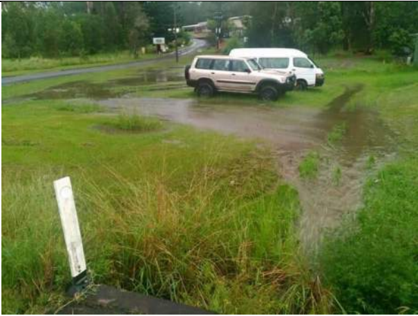
Photograph 8: Looking North up Hospital Road towards hospital. Photo taken at upstream inlet of culvert which passes underneath Woodenbong Road
