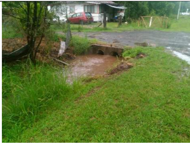
Photograph 4: Piped culverts underneath Post Office Ln. Looking South
