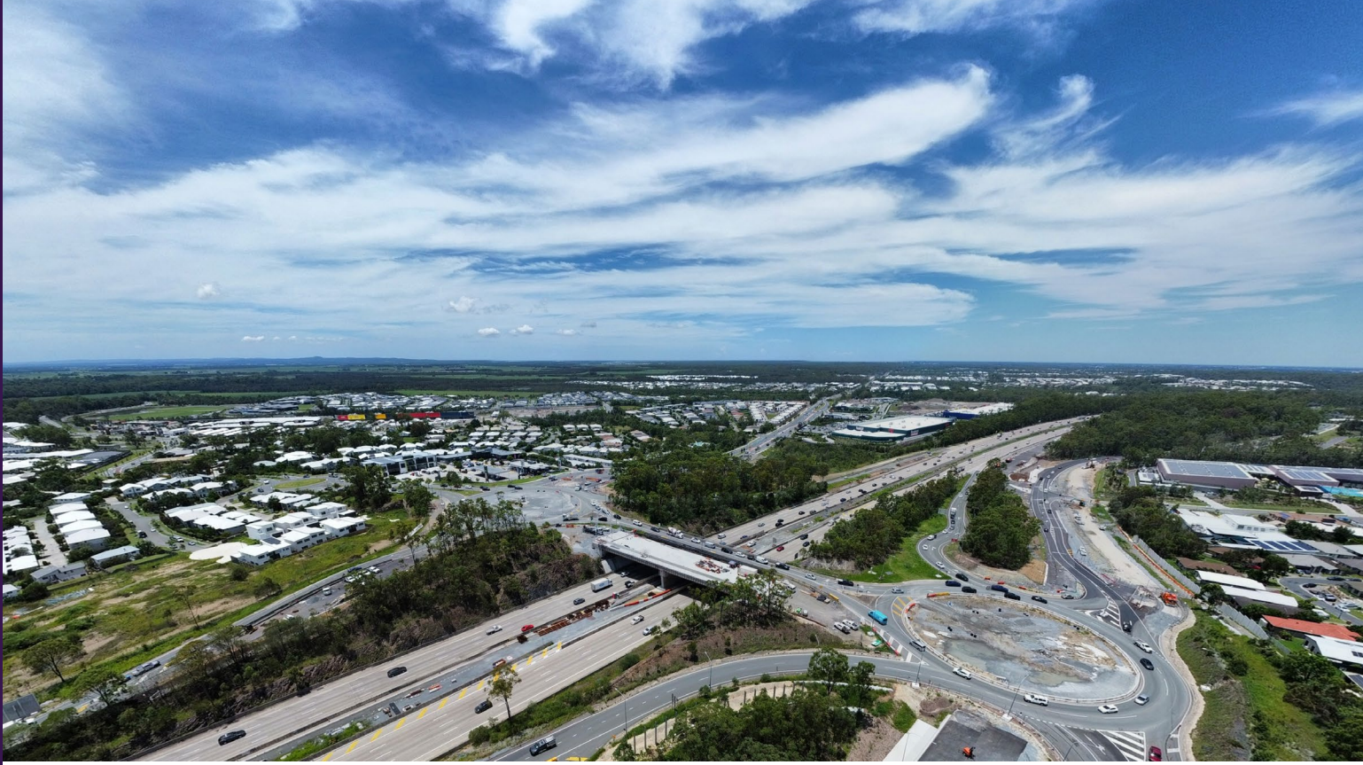
Pacific Highway (M1) Pimpama Interchange (Exit 49) - Gold Coast, QLD, Australia.
