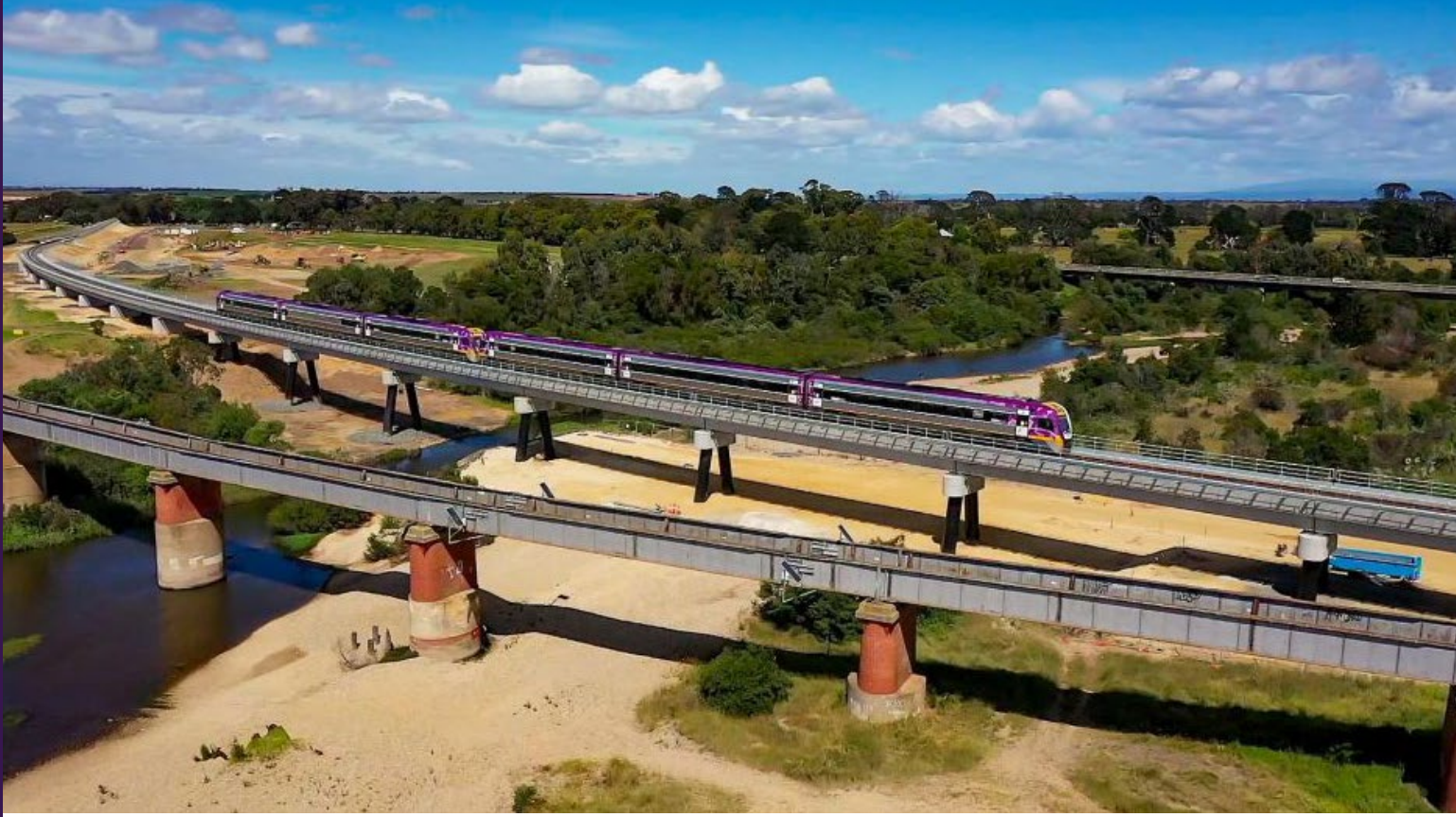
Avon River Bridge - Stratford, VIC, Australia.
