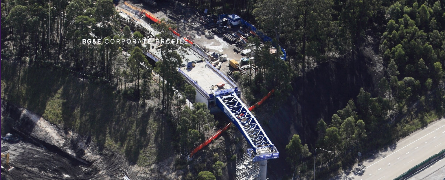
Hunter Expressway Flyover - Branxton, NSW, Australia.
