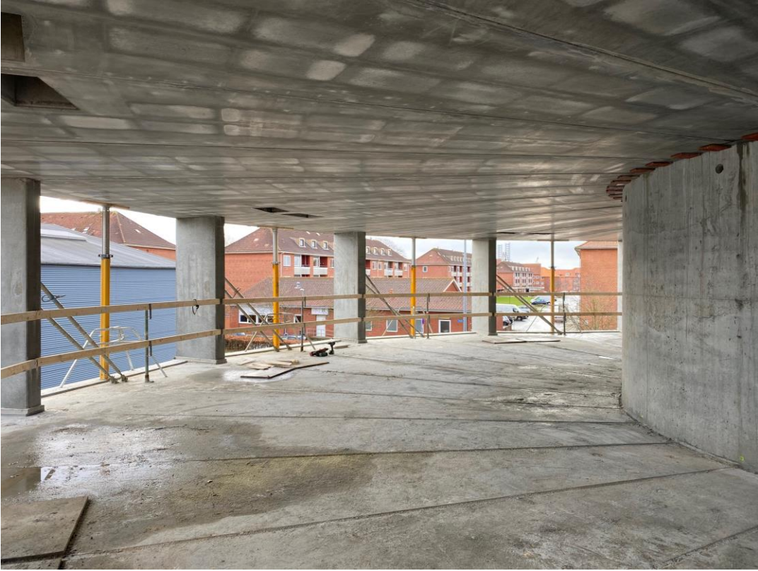
Figure 22. A Place To – Construction © A Place To / Abeo
