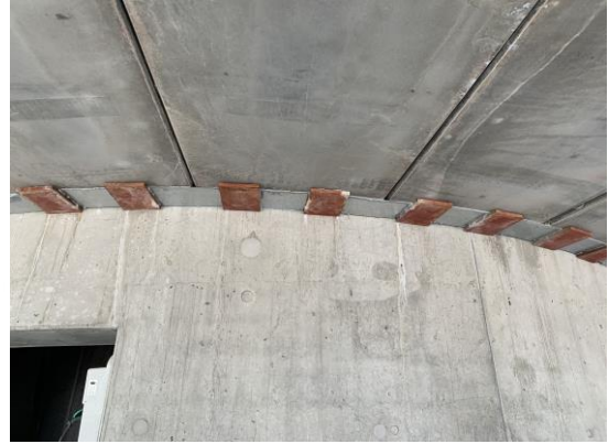
Figure 5. A Place To – Typical Floors of SL-slabs and steel corbel connection © Abeo / A Place To
