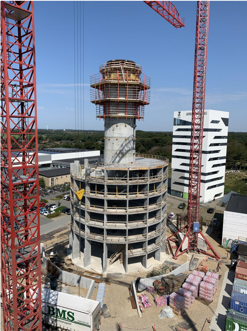
Figure 21. A Place To – Construction © A Place To / Abeo / PERI
