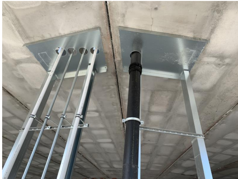
Figure 8. A Place To – MEP riser integration © Abeo / A Place To
