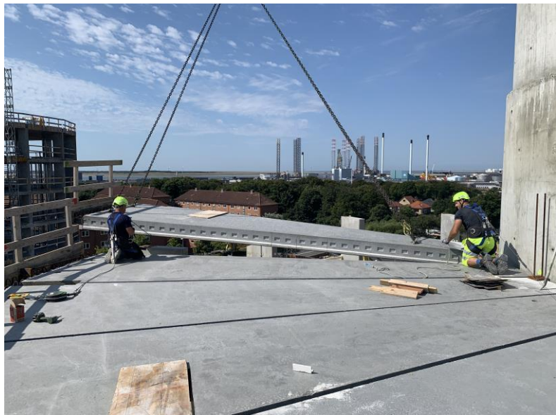
Figure 6. A Place To – SL-slabs during fabrication and installation © Abeo / A Place To
