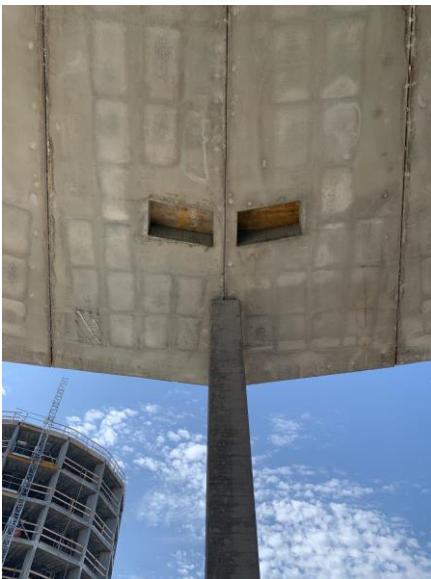
Figure 8. A Place To – MEP riser integration © Abeo / A Place To
