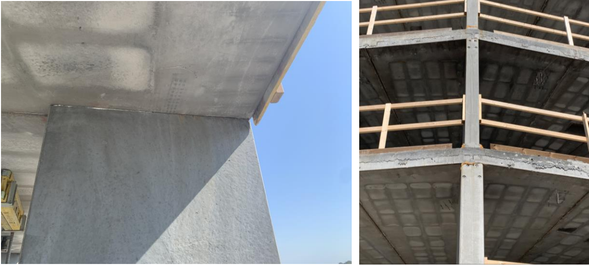
Figure 10. A Place To – Columns / SL-slab / Ring beam connection © A Place To
