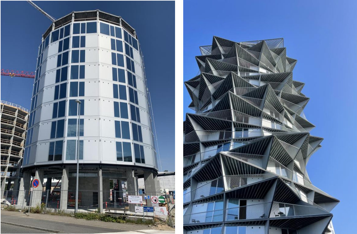
Figure 19. A Place To – Façade / Balcony installation © HSHansen / A Place To
