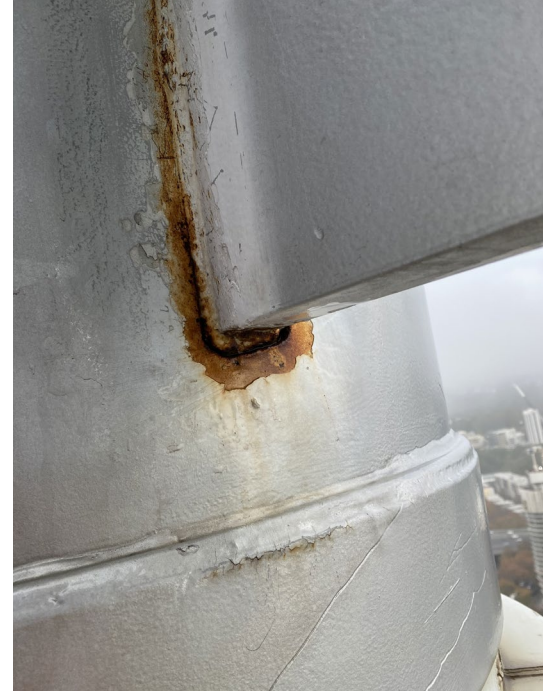
Assessment of steel rakers for recladding works for Central Park – Sydney, NSW, Australia.
