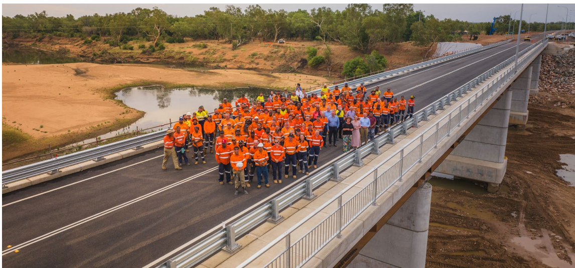
New Fitzroy River Bridge - Kimberley, WA, Australia
