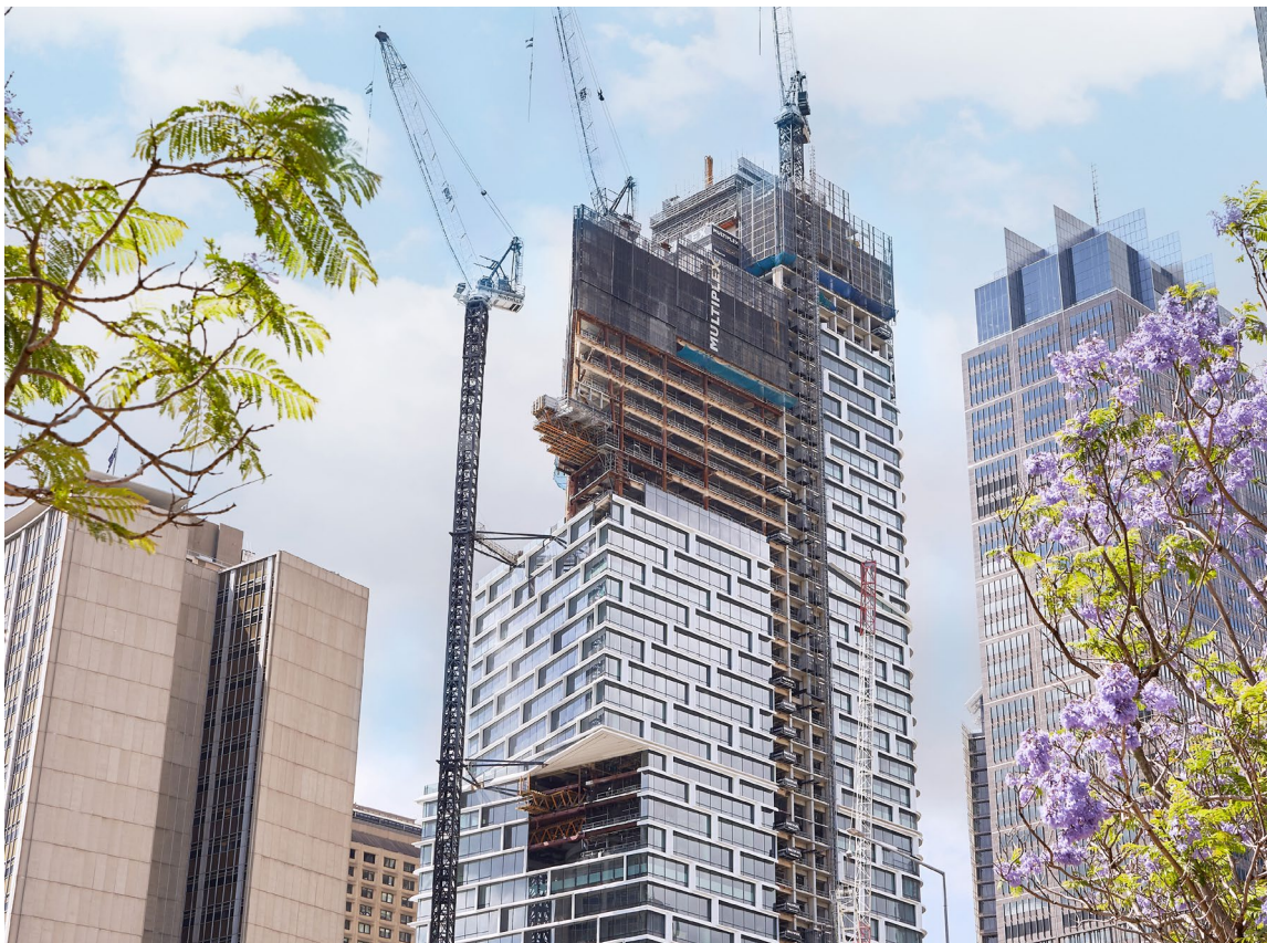
Quay Quarter Tower – Sydney, NSW, Australia
