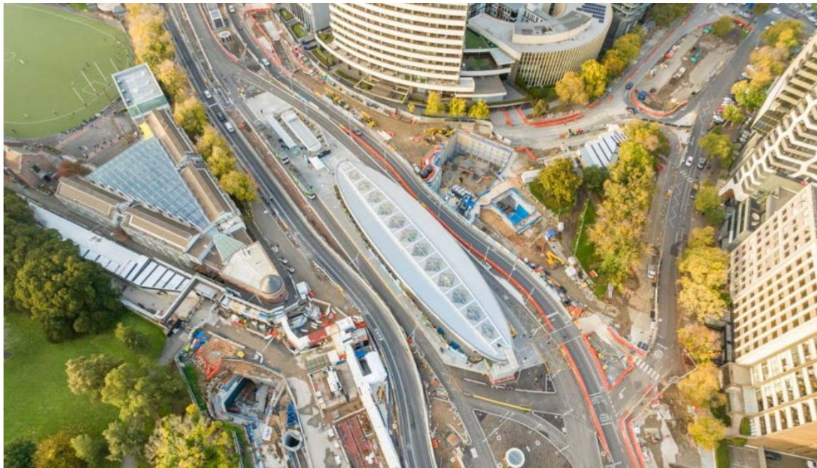
Melbourne Metro – Melbourne, VIC, Australia.
