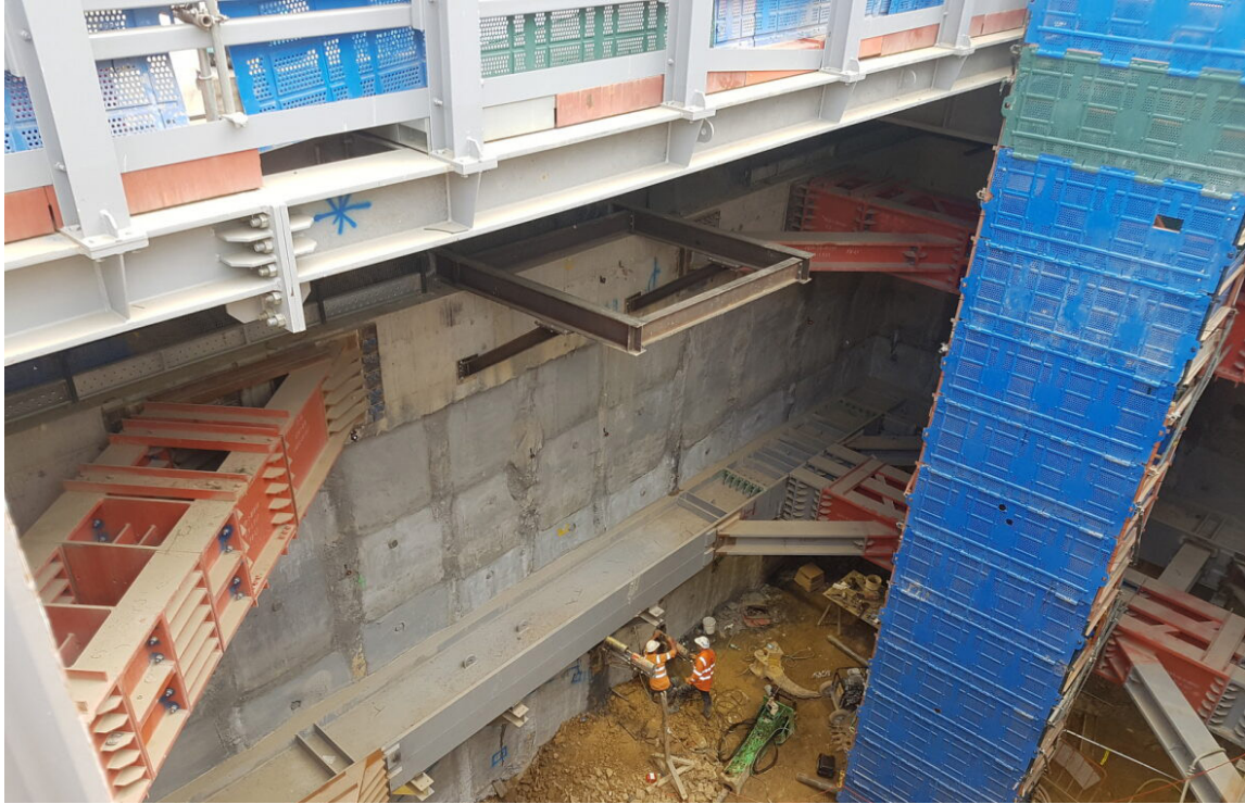
Melbourne Metro Flinders Link - Dive Structure - Melbourne, VIC, Australia.
