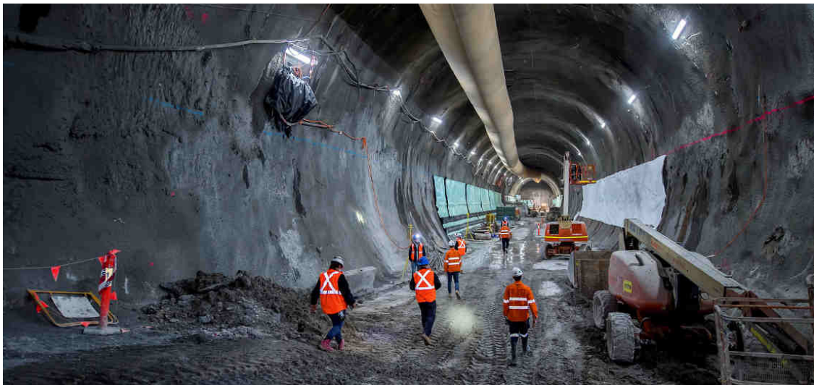
Sydney Metro City and Southwest - Sydney, NSW, Australia.
