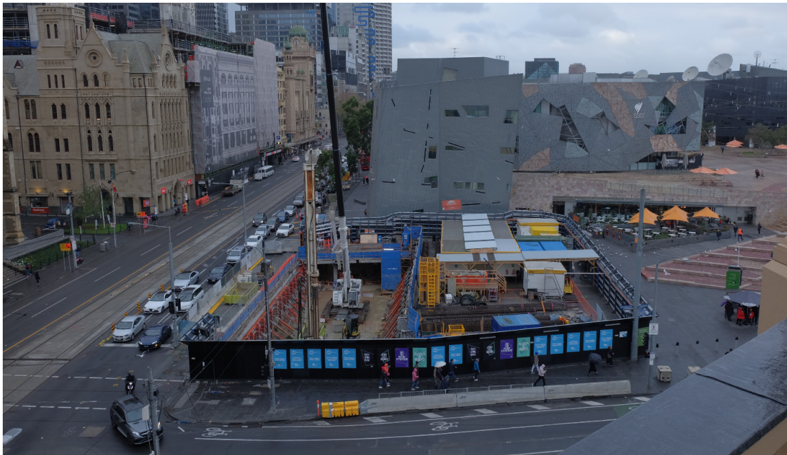
Melbourne Metro Federation Square - Temporary Works - Melbourne, VIC, Australia.
