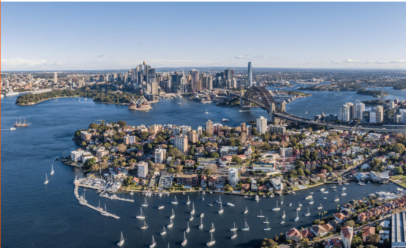
Western Harbour Tunnel – Sydney, NSW, Australia.
