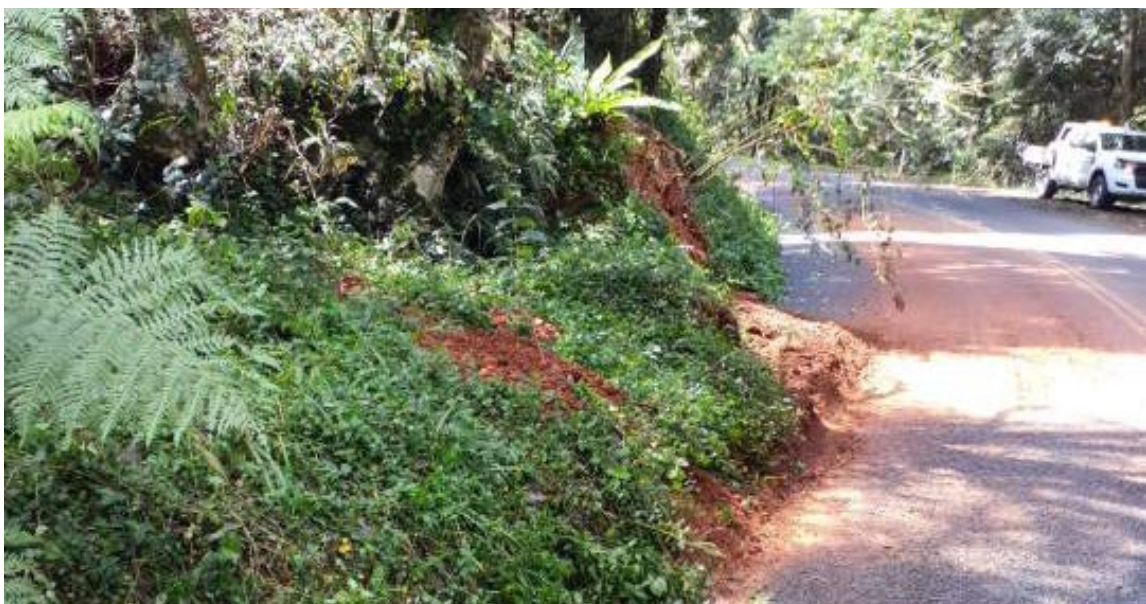
Flood Reconstruction Works, 2023 - Southern QLD, Australia.
