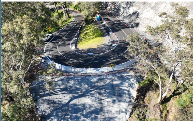
Flood Reconstruction Works, 2022 - Southern QLD, Australia.
