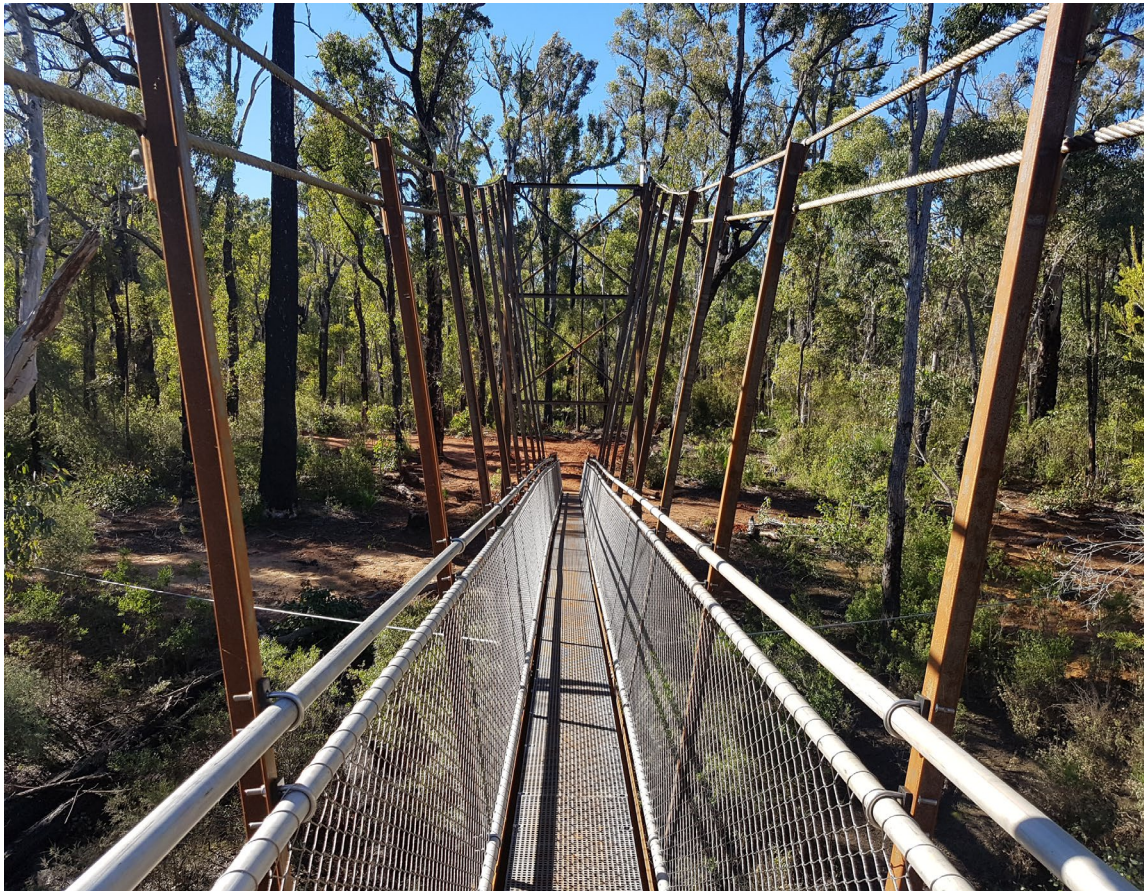
Bilya Djena Bidi Footbridge - Murray River, WA, Australia.
