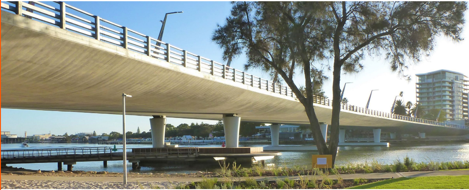
Pacific Highway Upgrade - Karuah Bypass - Sydney, NSW, Australia. Mandurah Estuary Bridge - Mandurah, WA, Australia.
