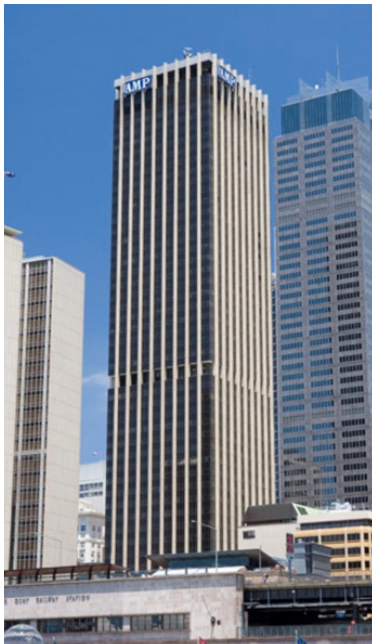
AMP Tower (constructed, 1976) - Sydney, NSW, Australia.
