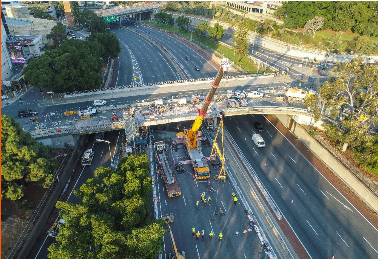
Hay Street Bridge – Perth, WA, Australia.
