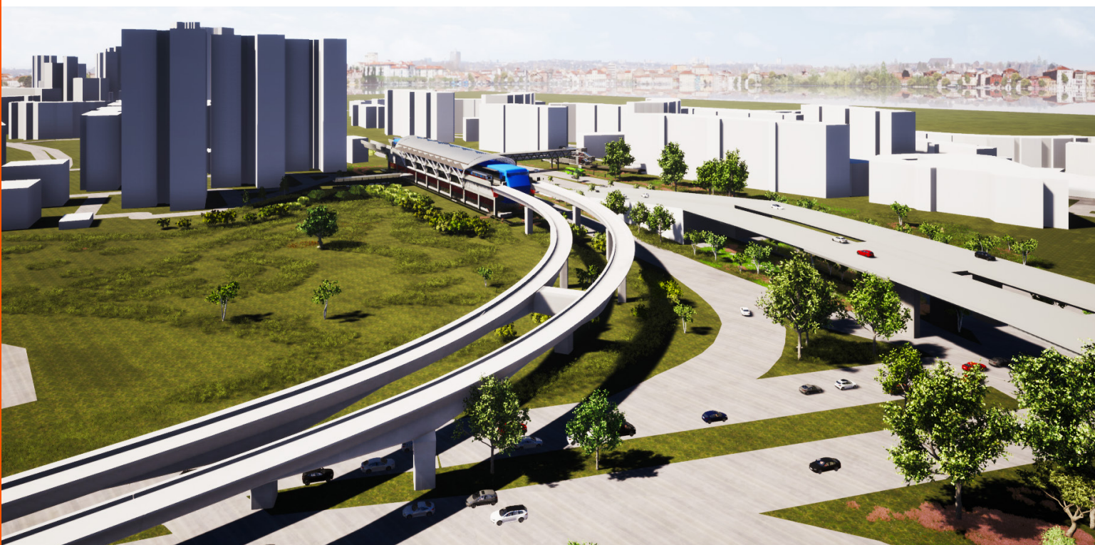
JRL 105 & 106 Rail Viaduct – Singapore, South East Asia.
