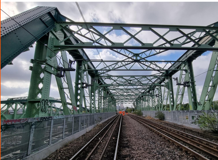
HS2 – SCS JV Asset Protection Framework – London, UK.
