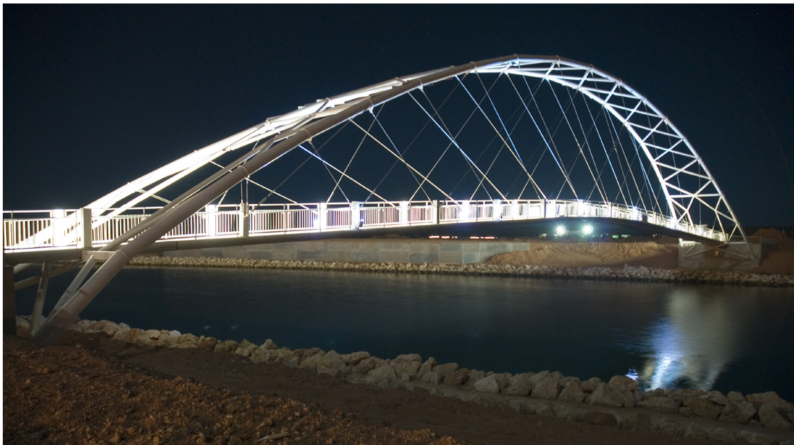
Exmouth Marina Footbridge – Exmouth, WA, Australia.
