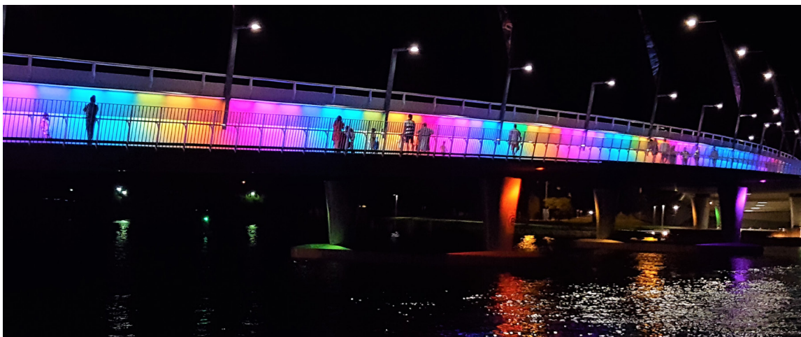
Mandurah Traffic Bridge – Mandurah, WA, Australia.
