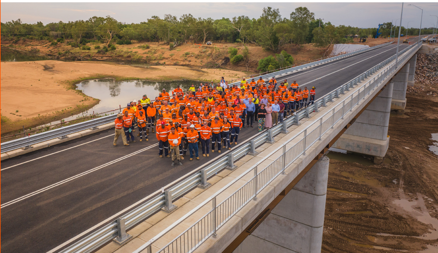
New Fitzroy River Bridge – Kimberley, WA, Australia.
