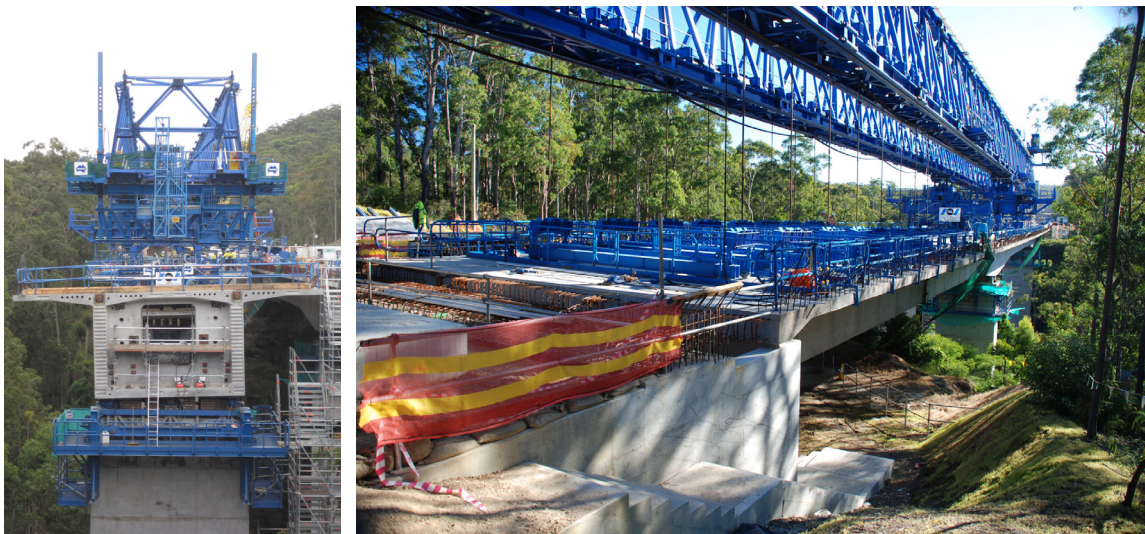
Hunter Expressway Flyover – Branxton, NSW, Australia.
