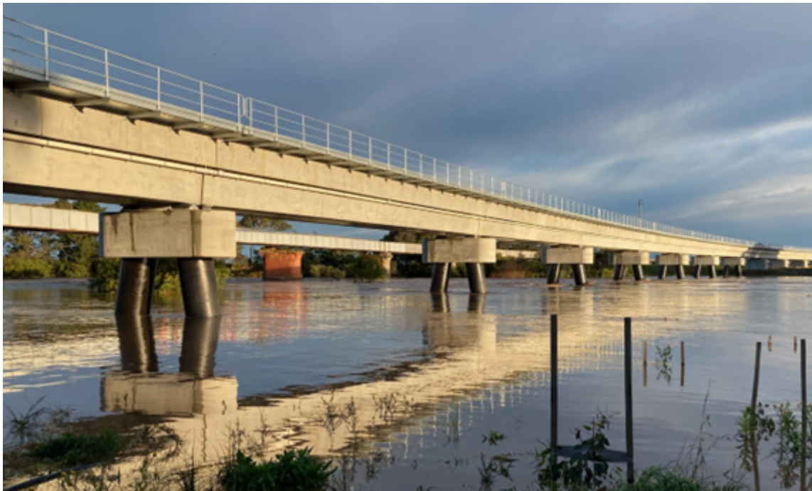
Avon River Bridge – Stratford, VIC, Australia.
