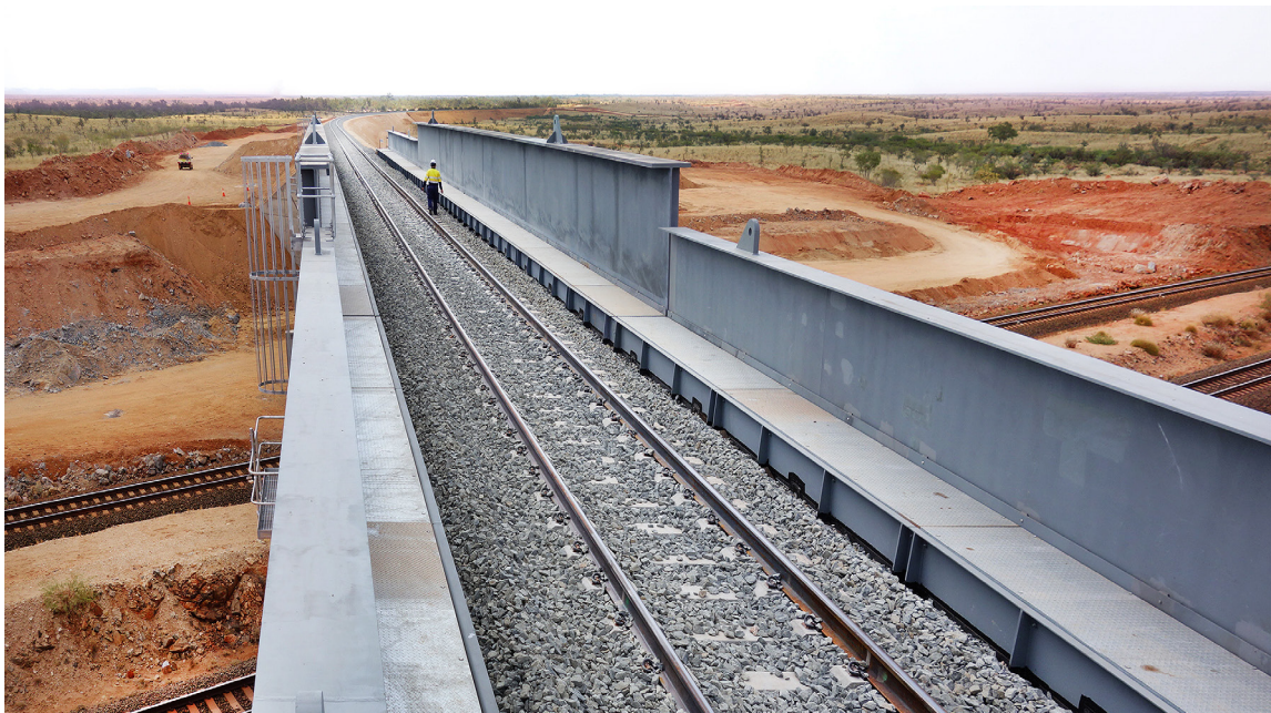
Roy Hill Railway Bridges – Pilbara Region, WA, Australia.
