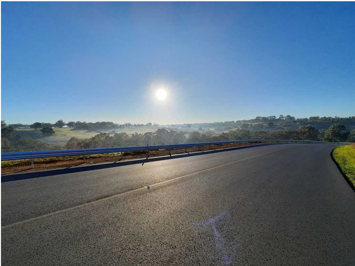
Exford & Greigs Road Bridges - Melton, VIC, Australia.
