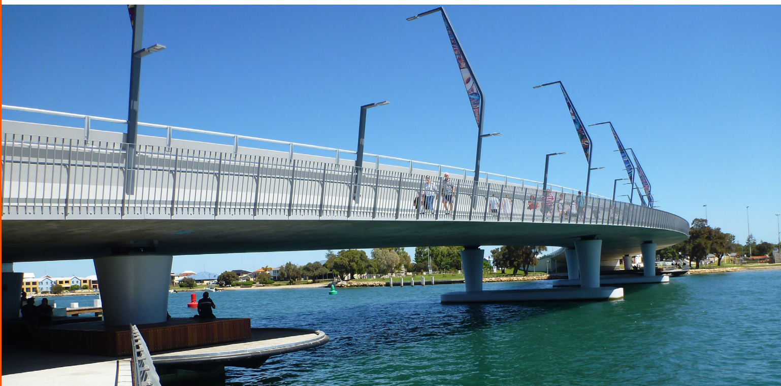
Mandurah Traffic Bridge – Mandurah, WA, Australia.
