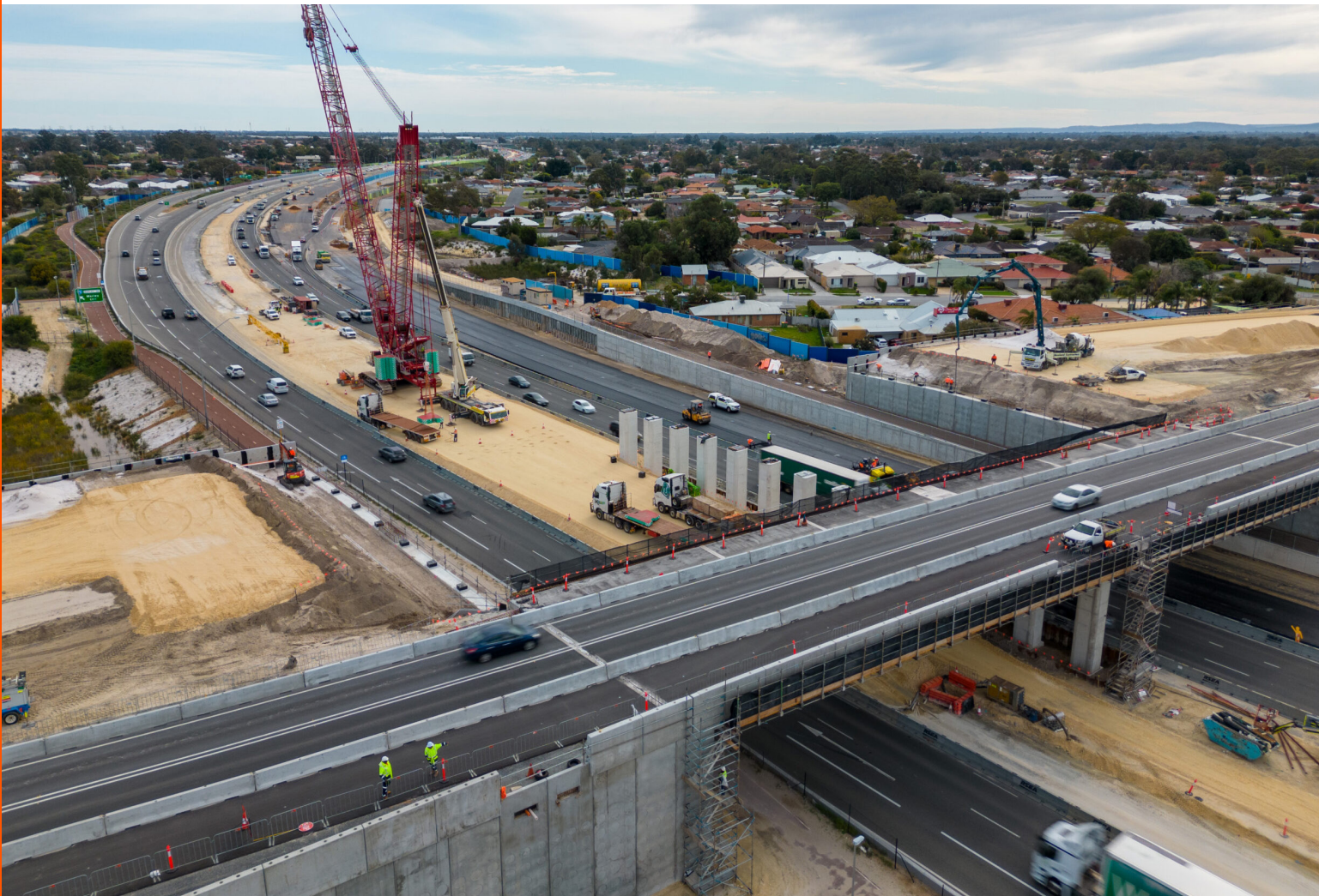
Tonkin Gap Project – Perth, WA, Australia.
