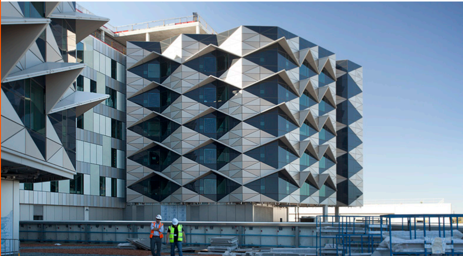
Fiona Stanley Hospital – Perth, WA, Australia.
