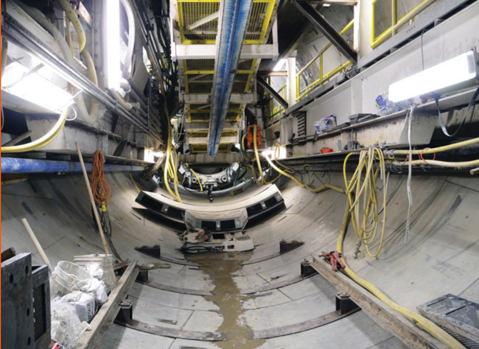
Sydney Metro - Western Sydney Airport Station - Sydney, NSW, Australia.
