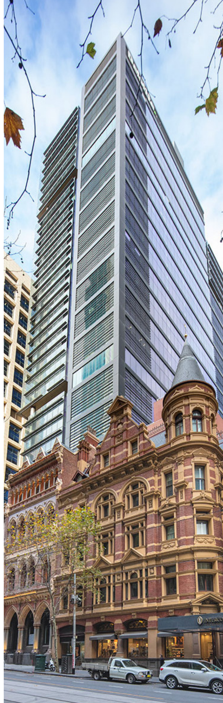
Olderfleet - Melbourne, VIC, Australia
