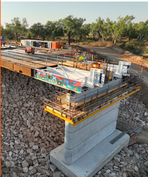
New Fitzroy River Bridge – Kimberley, WA, Australia.
