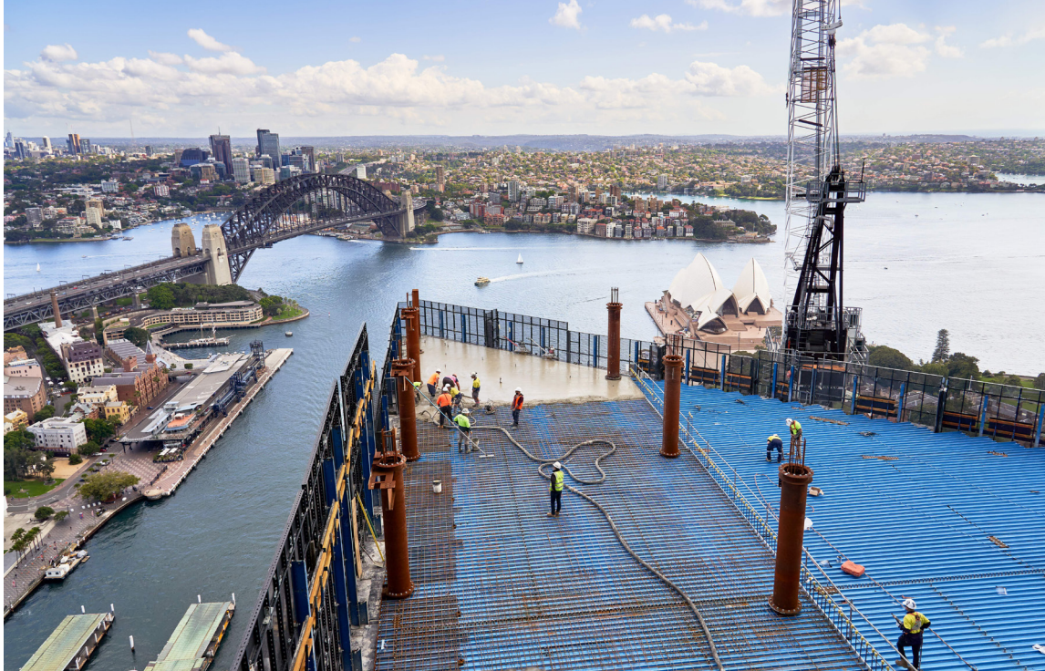
Quay Quarter Tower – Sydney, NSW, Australia.
