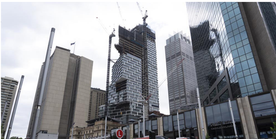
Quay Quarter Tower – Sydney, NSW, Australia.
