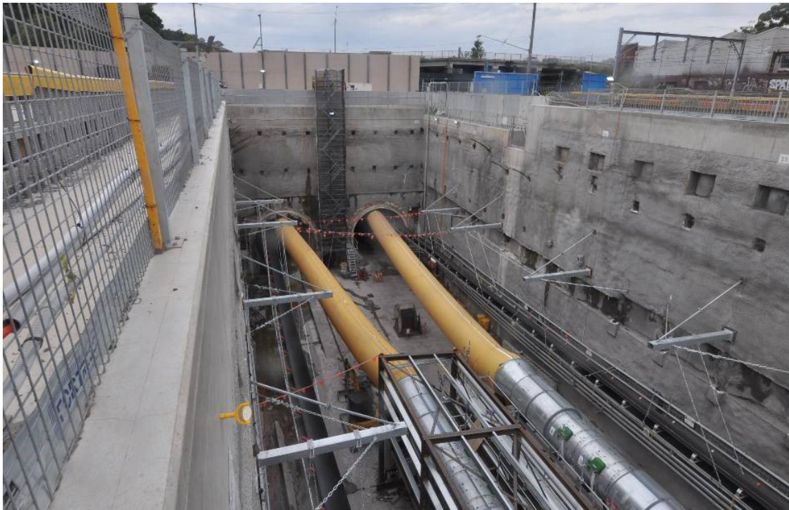
Sydney Metro City & Southwest (SMCSW) - Sydney, NSW, Australia.
