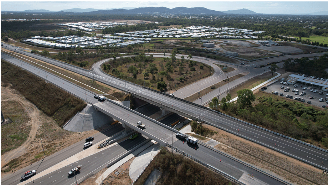
Townsville Ring Road: Stage Five - Townsville, QLD, Australia.
