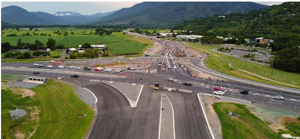
Smithfield Bypass – Cairns, QLD, Australia.
