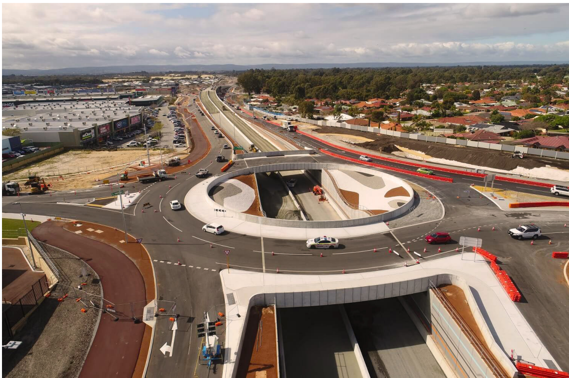
Armadale Road & North Lake Road – Perth, WA, Australia.
