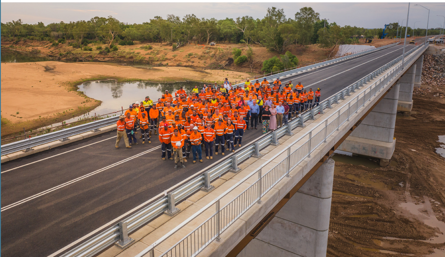
New Fitzroy River Bridge – Kimberley, WA, Australia.
