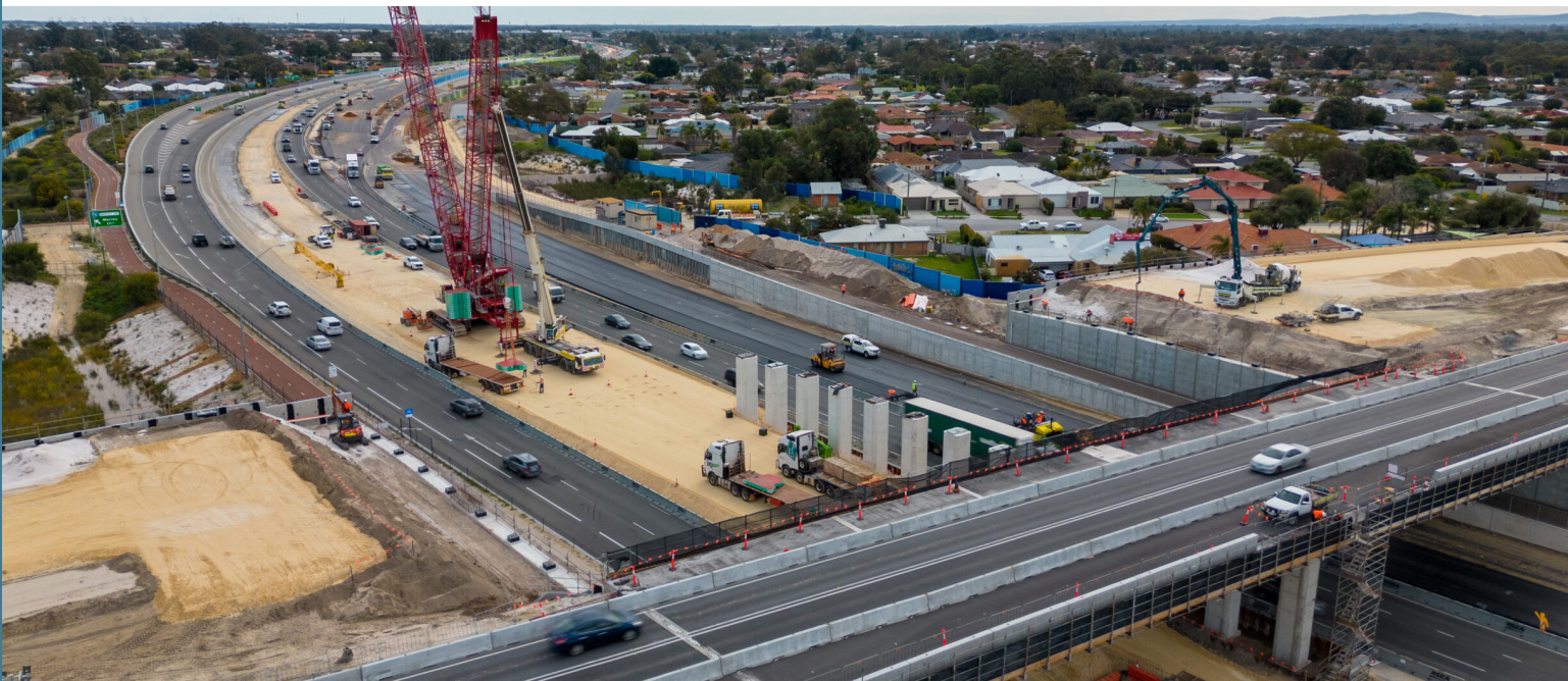
Tonkin Gap Project - Perth, WA, Australia.
