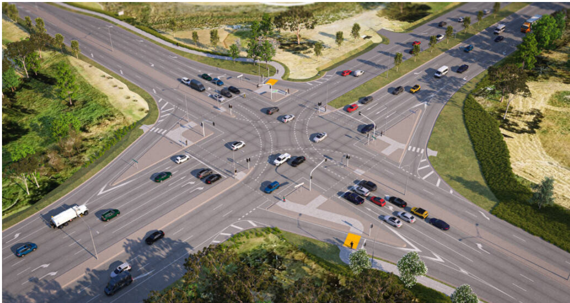
Western Port Highway Upgrade – Melbourne, VIC, Australia.
