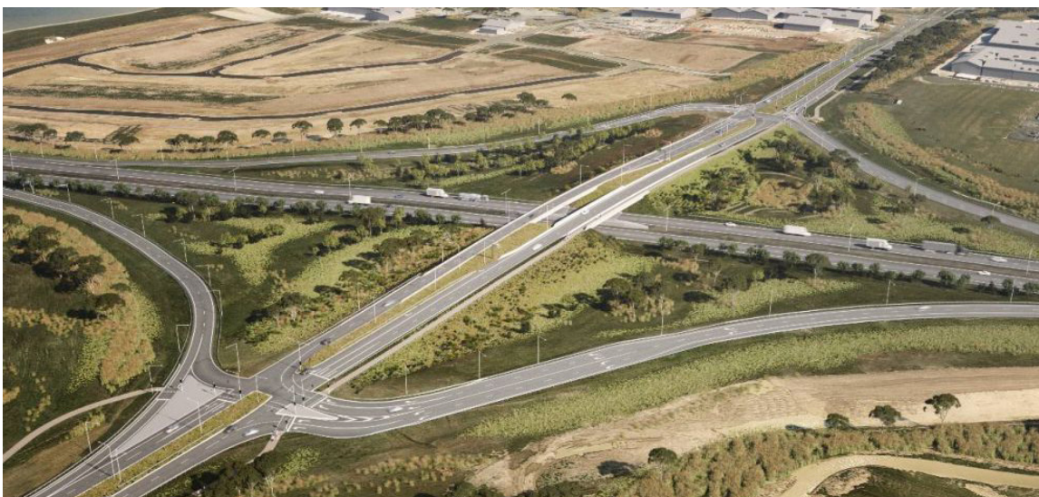
Pakenham Roads Upgrade - Pakenham, VIC, Australia.
