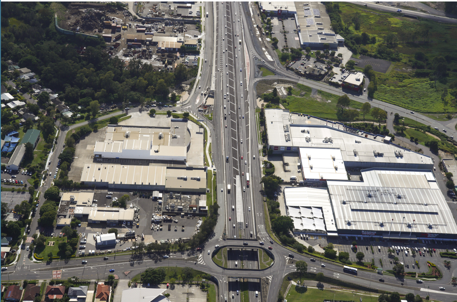
Ipswich Motorway Upgrade Project - Stage One: Rocklea to Darra - Brisbane, QLD, Australia.
