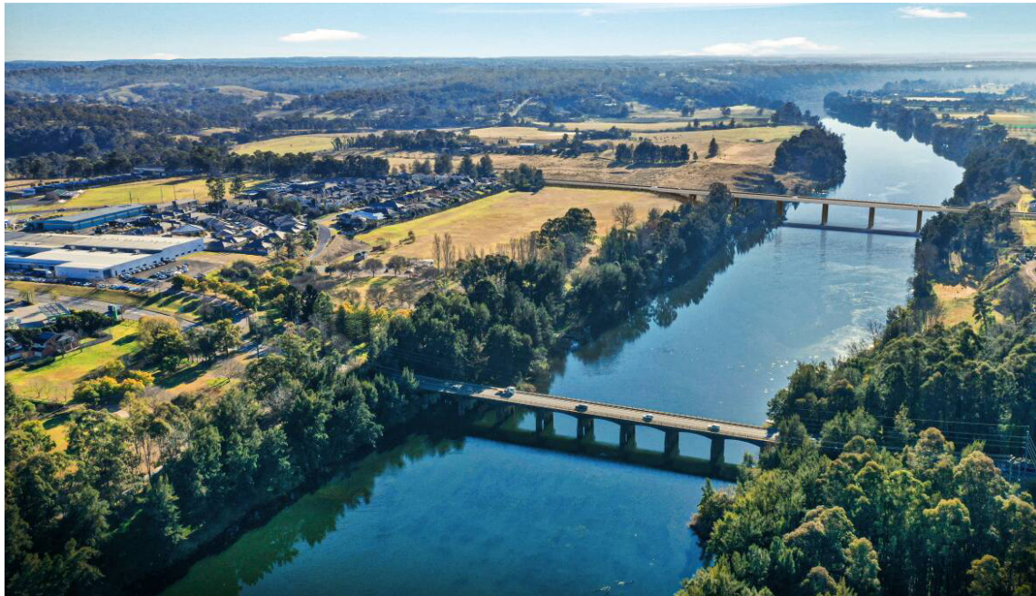
New Richmond Bridge: Stage One - The Driftway - Richmond, NSW, Australia.
