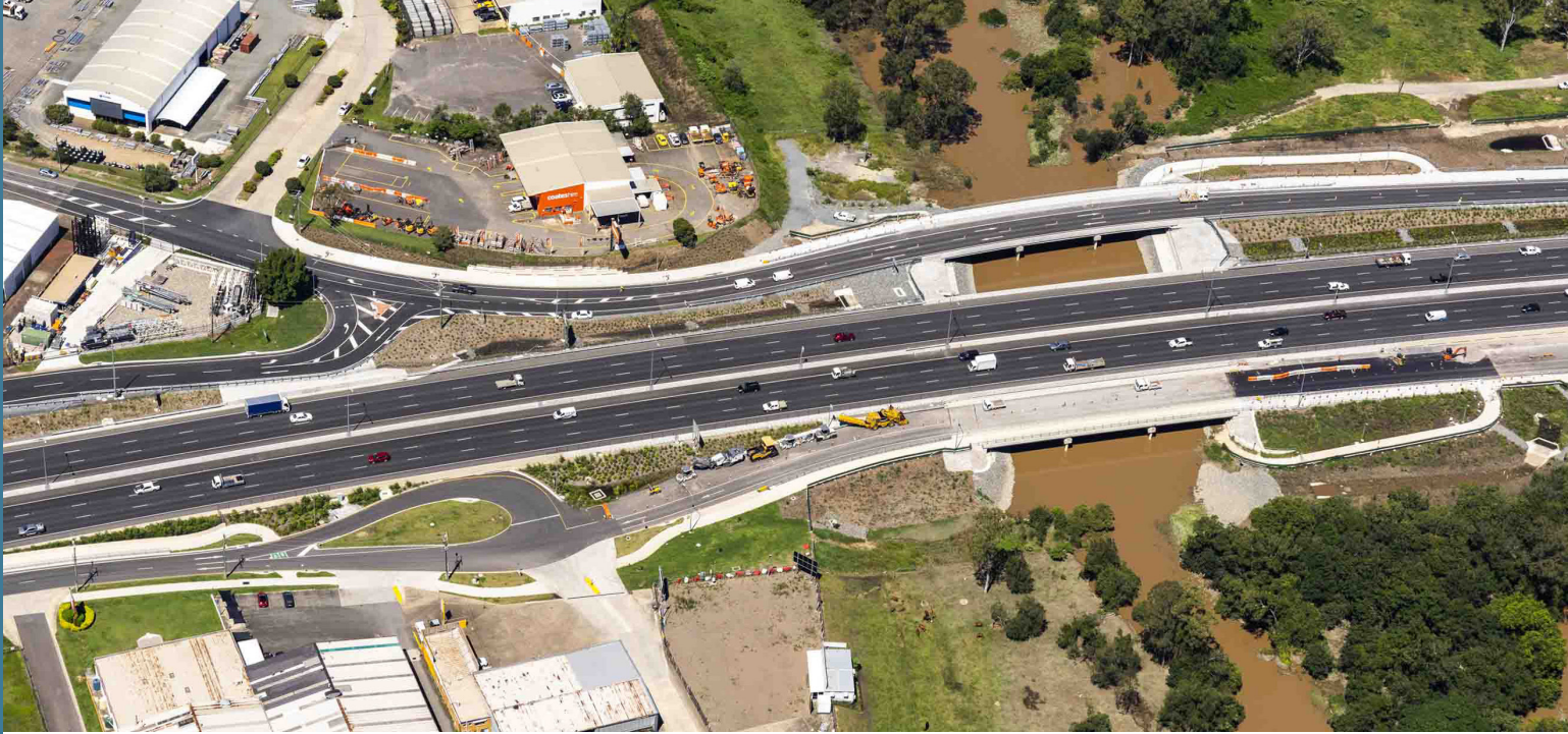
Pacific Highway Upgrade, Woolgoolga to Ballina - Portion A - North Coast, NSW, Australia.
