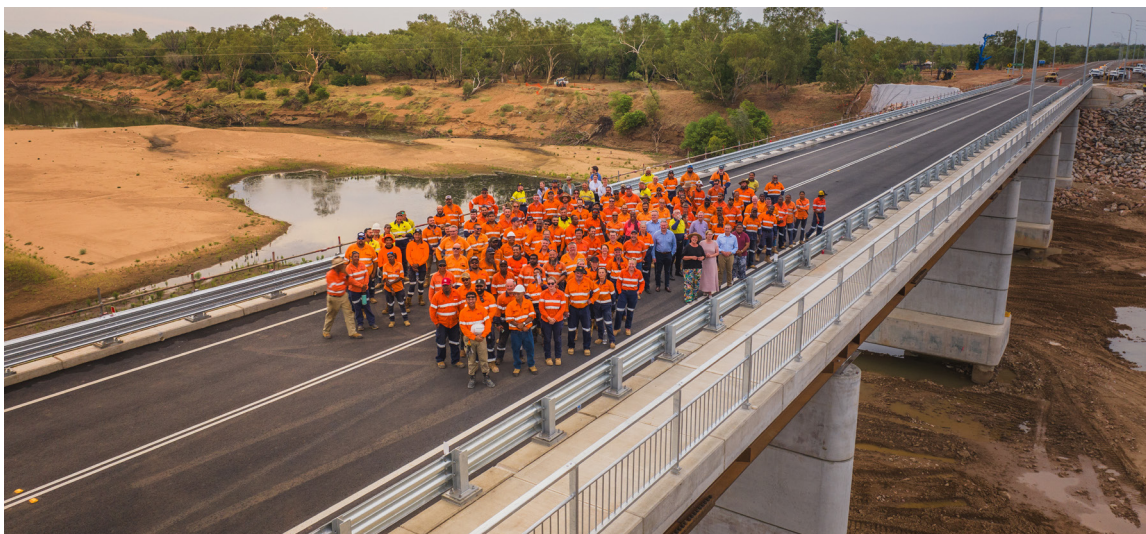
New Fitzroy River Bridge - Kimberley, WA, Australia
