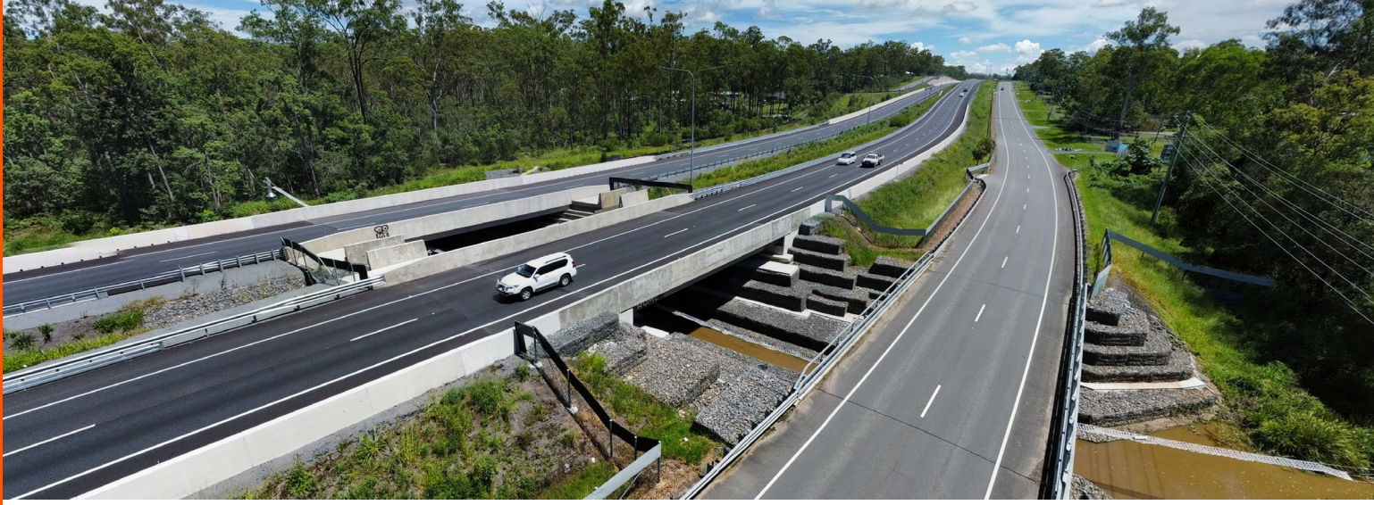
Mount Lindesay Highway, Stoney Camp Road to Chambers Flat - Brisbane, QLD, Australia.
