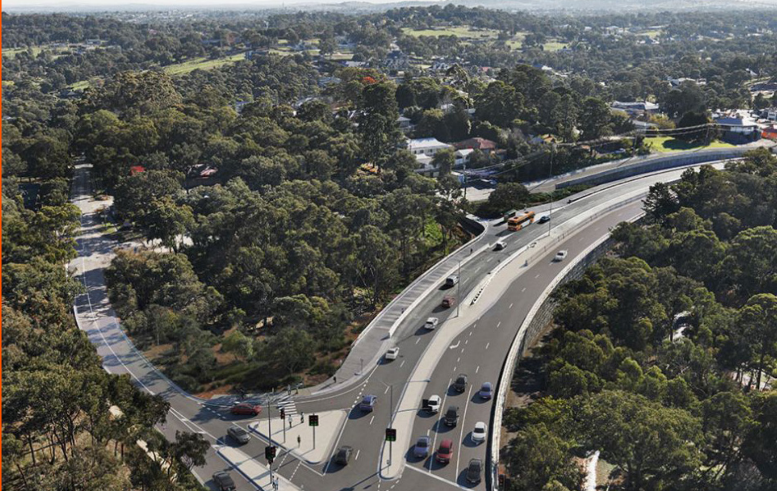
Yan Yean Road Upgrade (Stage 1) - Melbourne, VIC, Australia.
