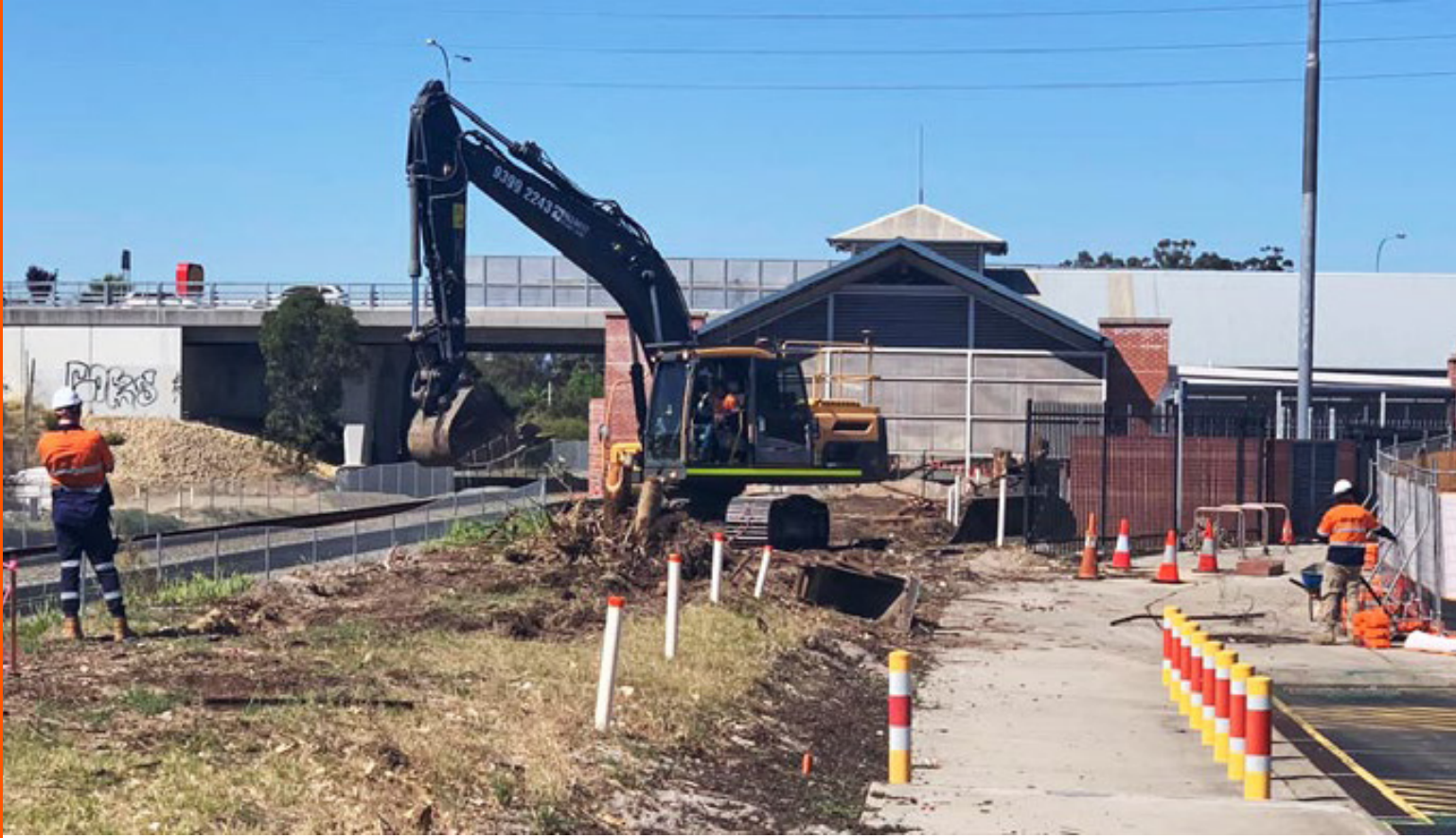
METRONET – Thornlie to Cockburn Rail Upgrade – Perth, WA, Australia.
