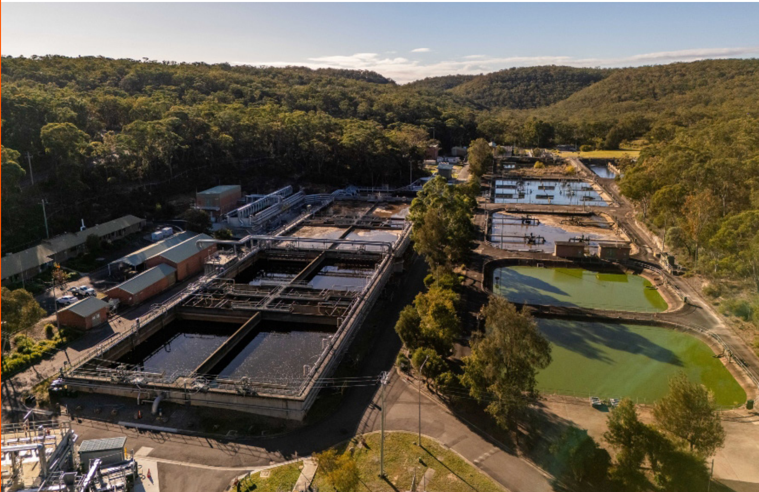
Winmalee Sewerage Treatment Plant Upgrade - Blue Mountains, NSW, Australia.
