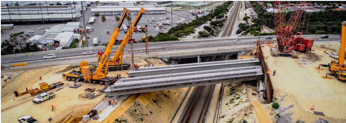
METRONET – Thornlie to Cockburn Rail Upgrade – Perth, WA, Australia.
