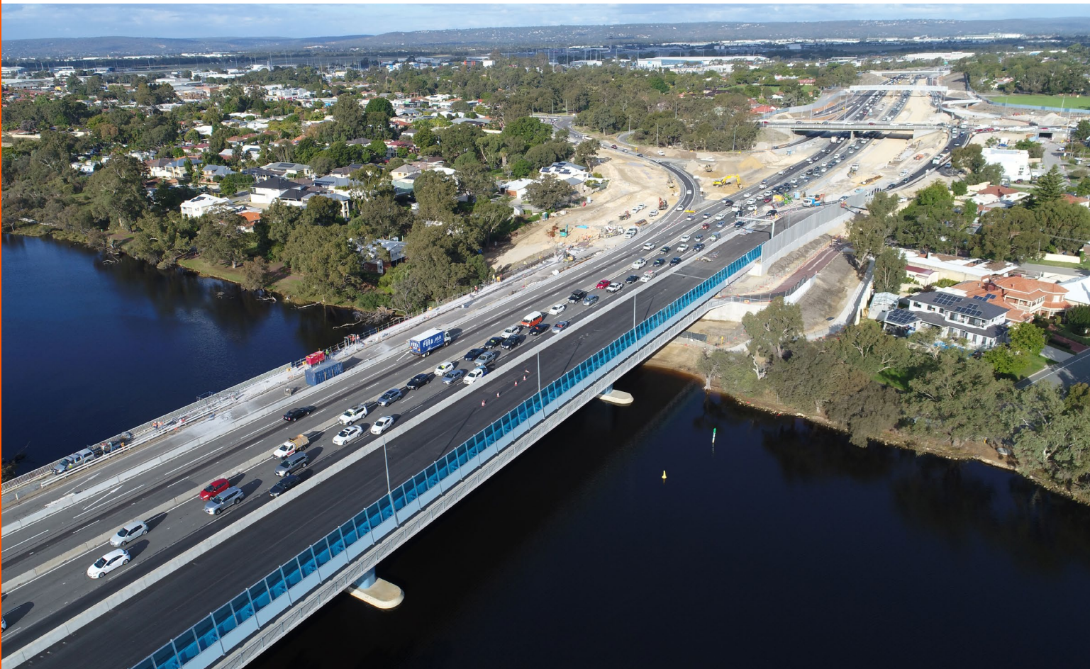
Tonkin Gap Project – Perth, WA, Australia.
