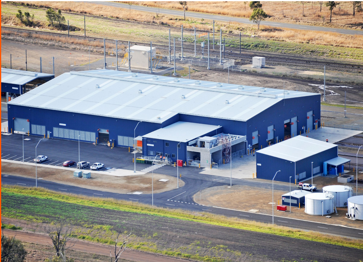
Nebo Train Maintenance Facility – Brisbane, QLD, Australia.
