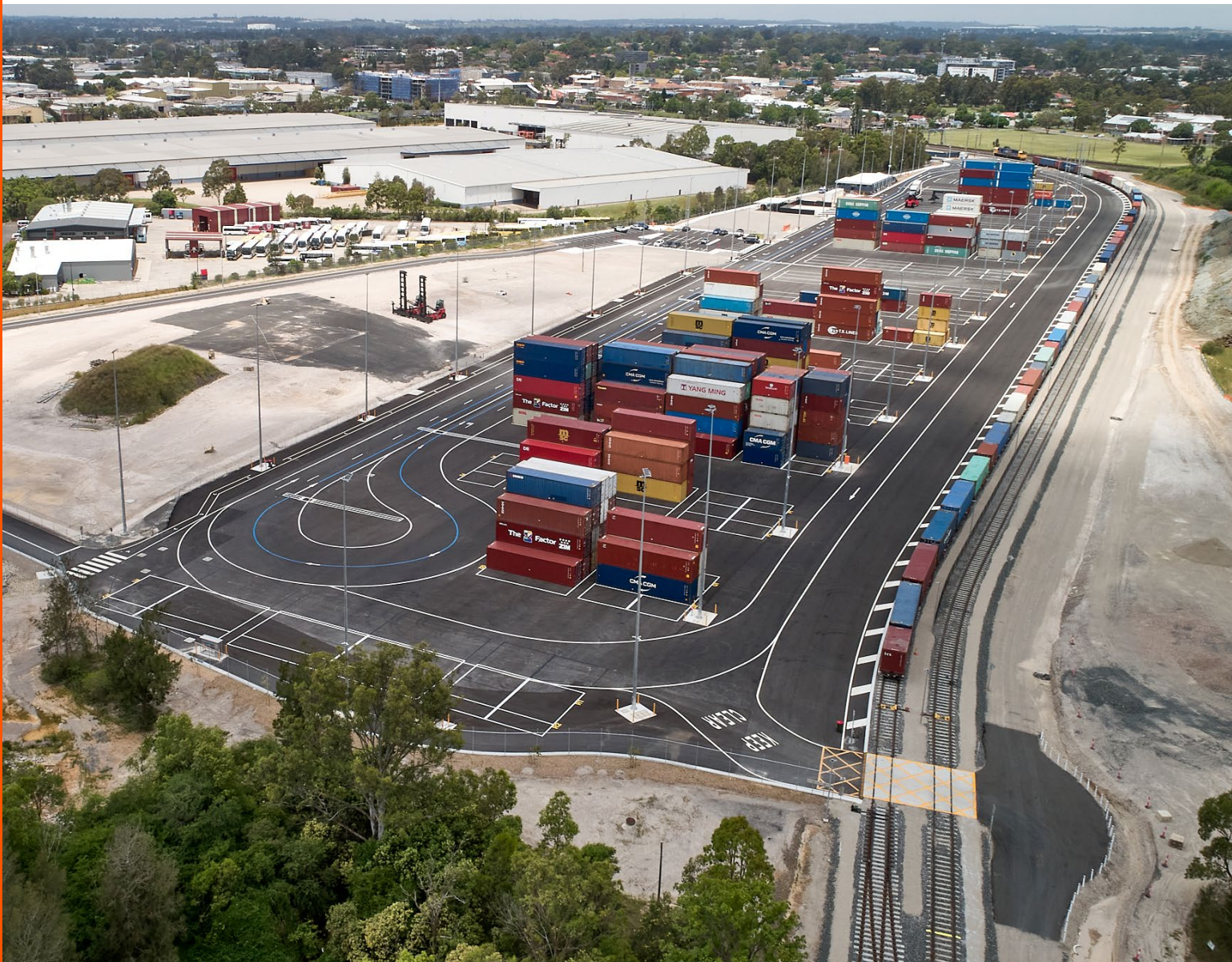
St Mary's Freight Hub – Sydney, NSW, Australia.
