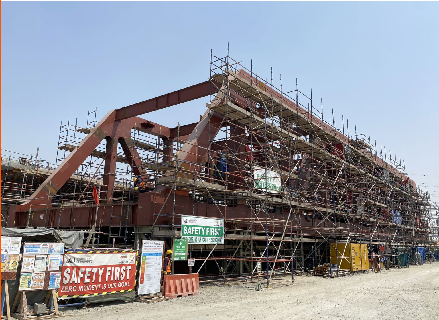
Etihad Rail Network Viaducts, Stage 2 – Abu Dhabi, United Arab Emirates.
