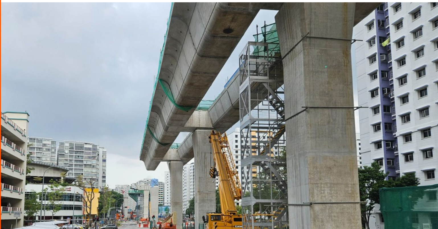
JRL 105 & 106 Rail Viaduct – Singapore, South East Asia.
