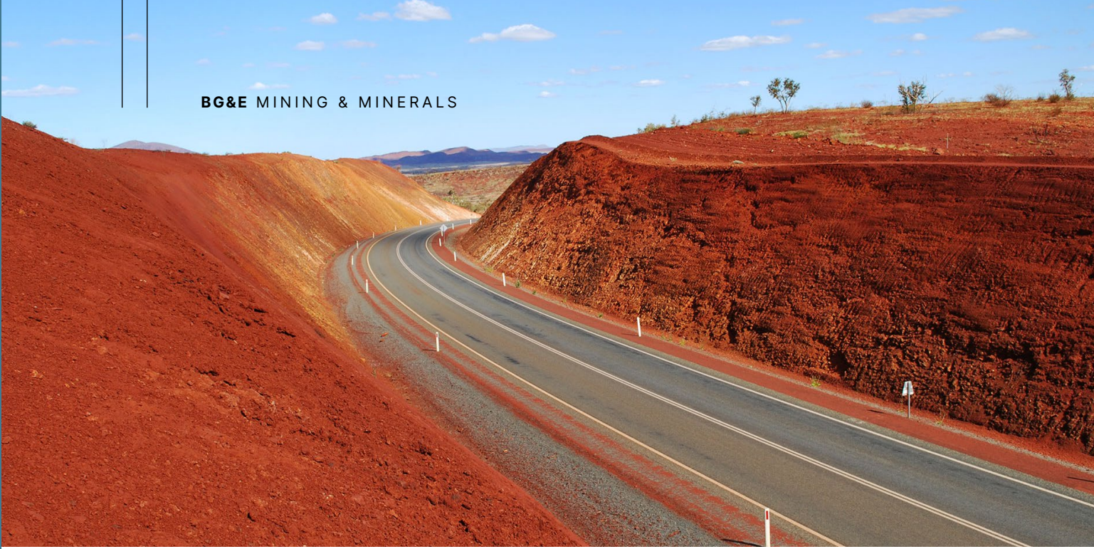
Brockman 4 Project: Brockman 2 to Brockman 4 Access Road - Pilbara, WA, Australia.
