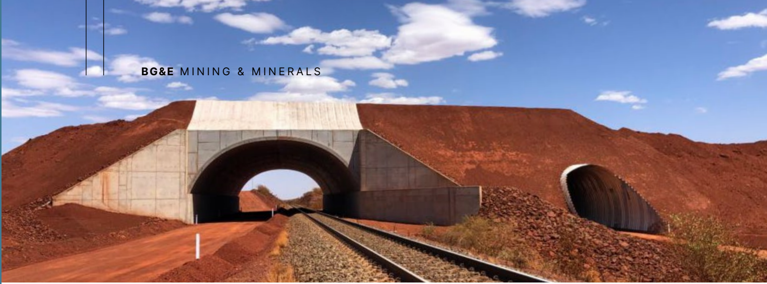
Abrolhos Overpass - Pilbara, WA, Australia.
