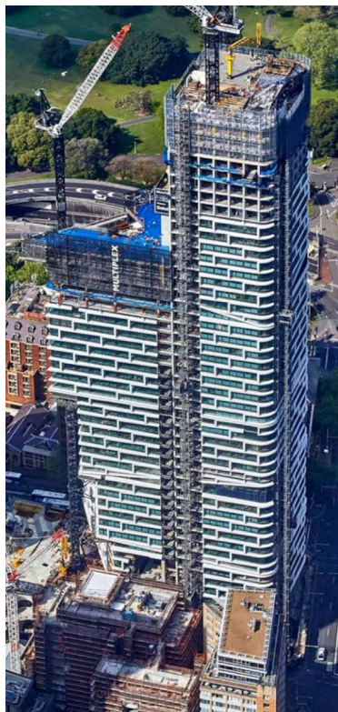
Quay Quarter Tower (in construction, 2021) — Sydney, NSW, Australia.
