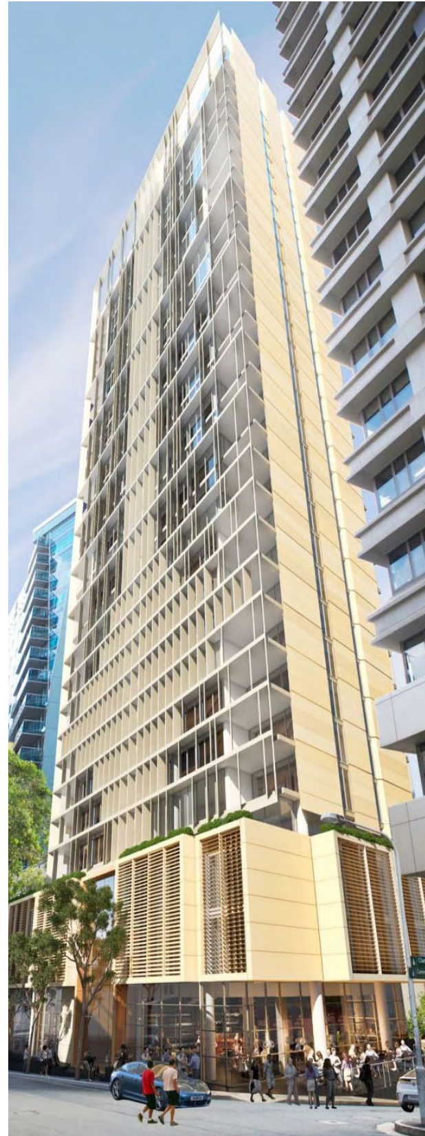
9-25 Commonwealth Street, Edition Residences — Sydney, NSW, Australia. Structural Engineering services provided.
