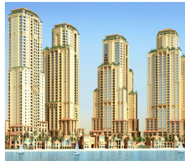
Jumeirah Beach Residences Structural Dubai, United Arab Emirates.
