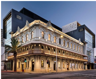
Melbourne Hotel Structural Perth, WA, Australia.
