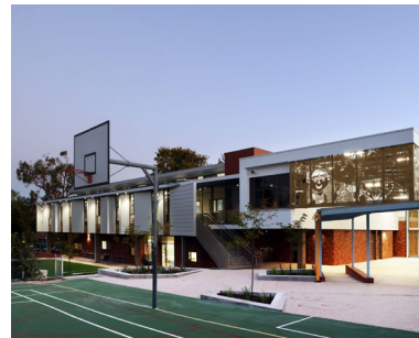
Scarborough Primary School Redevelopment Structural | Civil Scarborough, WA, Australia.
