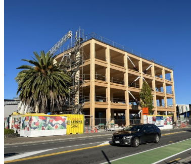
211 High Street Structural | Timber Christchurch, New Zealand.
