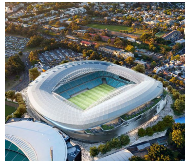
Moore Park Stadium Construction Engineering Sydney, NSW, Australia.
