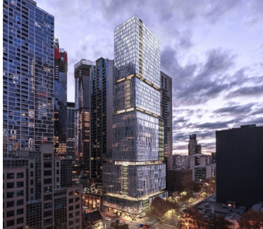
600 Lonsdale Street Façade Melbourne, VIC, Australia.
