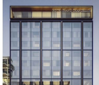
Hotel Grand Chancellor Construction Engineering Nedlands, WA, Australia.
