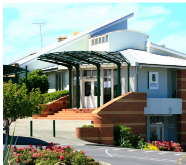
Lynfield College Façade Auckland, New Zealand.
