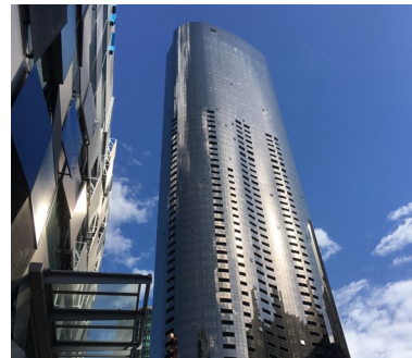
Prima Pearl Apartments (254m) Façade Melbourne, VIC, Australia.
