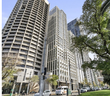
17 Spring Street Façade Melbourne, VIC, Australia.
