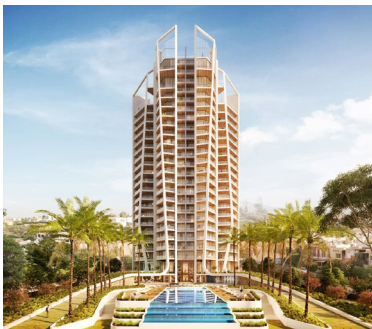
Sky Tower Structural | Construction Engineering Limassol, Cyprus.
