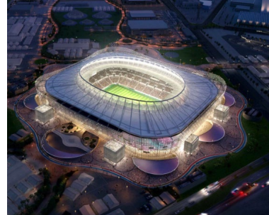
Al Rayyan Sports Club Stadium Structural Doha, Qatar.
