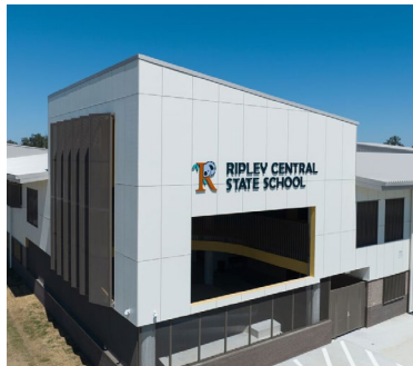
Ripley Central State School Structural Ipswich, QLD, Australia.
