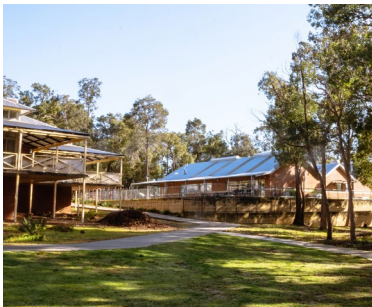
Roleystone Community College Structural | Civil | Timber Perth, WA, Australia.
