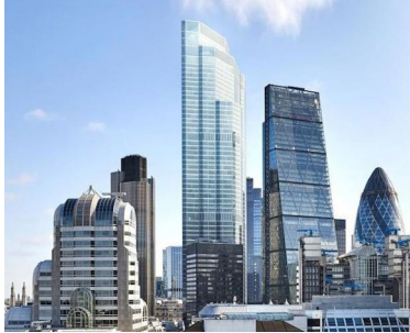
22 Bishopgate (278m) Construction Engineering London, United Kingdom.
