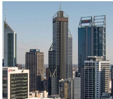
Central Park Tower Structural | Construction Engineering Perth, WA, Australia.
