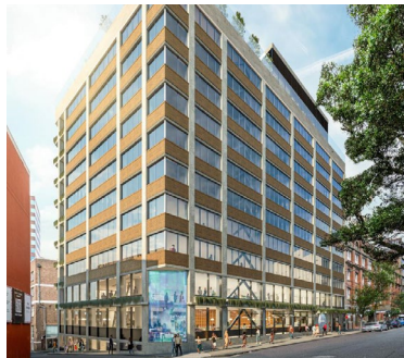
Canva Global Headquarters Structural | Construction Engineering Sydney, NSW, Australia.
