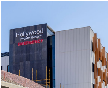
Hollywood Private Hospital South Block & Emergency Department Structural | Civil Nedlands, WA, Australia.
