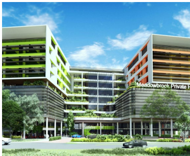
Meadowbrook Private Hospital — Australia Unity Health Precinct Structural | Civil Brisbane, QLD, Australia.
