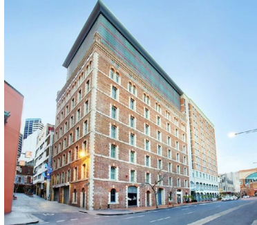
Holiday Inn Darling Harbour Structural Sydney, NSW, Australia.
