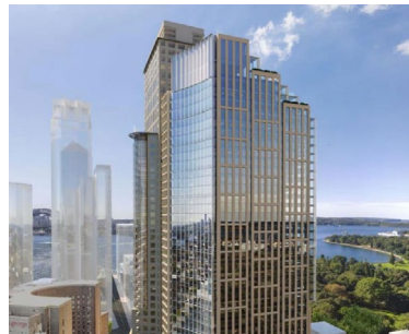
Chifley Tower (244m) Structural Sydney, NSW, Australia.
