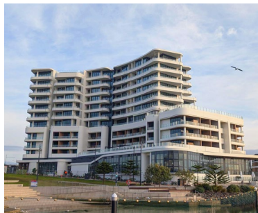
Shell Cove Harbour Hotel Structural Shell Harbour, NSW, Australia.
