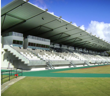
AK Reserve Stadium Structural Mount Claremont, WA, Australia.
