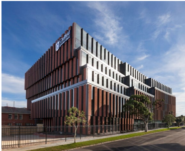
Caulfield Grammar School Façade Melbourne, VIC, Australia.
