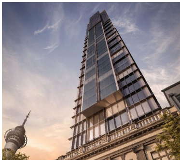
Hotel Indigo Construction Engineering Auckland, New Zealand.
