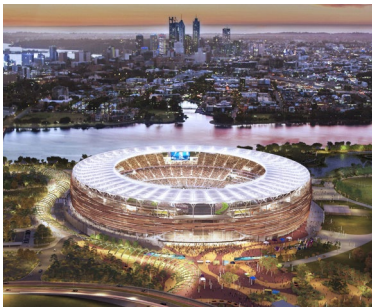
Optus Stadium Transport Projects Structural | Civil Burswood, WA, Australia.
