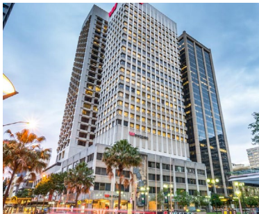
260 Queen Street Structural Brisbane, QLD, Australia.
