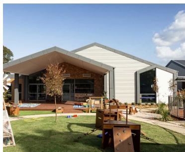
St Nicholas Early Education Lochinvar Structural | Civil Hunter Region, NSW, Australia.
