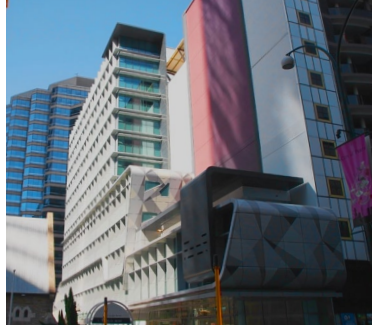
167 St Georges Terrace Structural | Civil Perth, WA, Australia.
