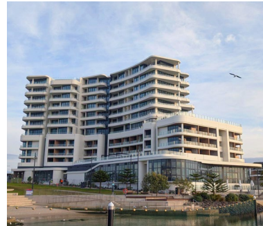
Shell Cove Harbour Hotel Structural Shellharbour, NSW, Australia.
