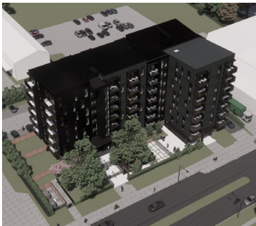
NC12 Apartments Structural | Construction Engineering Auckland, New Zealand.
