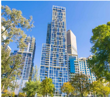
35 Spring Street Façade Melbourne, VIC, Australia.
