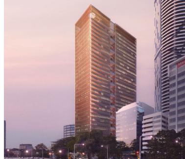
205 North Quay Façade Brisbane, QLD, Australia.
