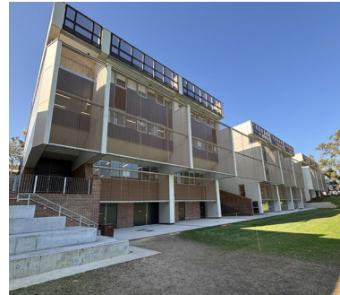
Carine Senior High School Structural Perth, WA, Australia.
