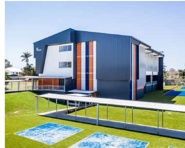
Cleveland State High School Structural Brisbane, QLD, Australia.
