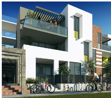
The Bottleyard Apartments Structural | Civil Leederville, WA, Australia.
