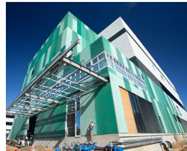
QEII Central Energy Plant Structural Nedlands, WA, Australia.
