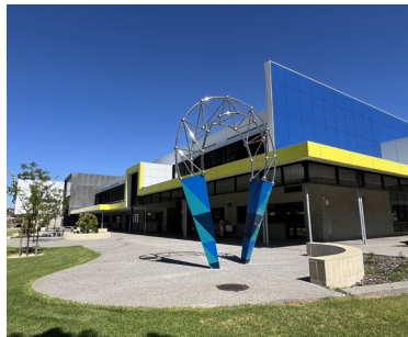
Rossmoyne Senior High School Structural | Civil Perth, WA, Australia.
