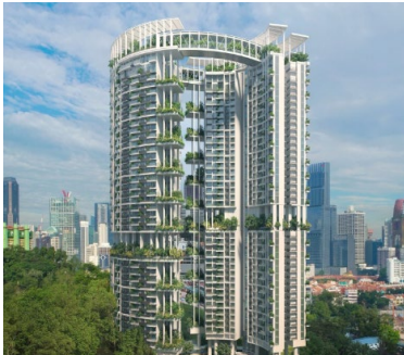
One Pearl Sky Bridge Construction Engineering Singapore.
