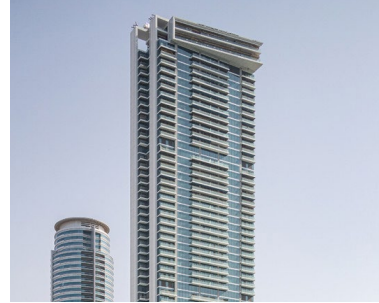
Vida Dubai Marina & Yacht Club (230m) Structural Dubai, United Arab Emirates.
