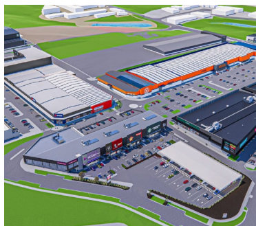
Kakano Centre Structural Peer Review Auckland, New Zealand.
