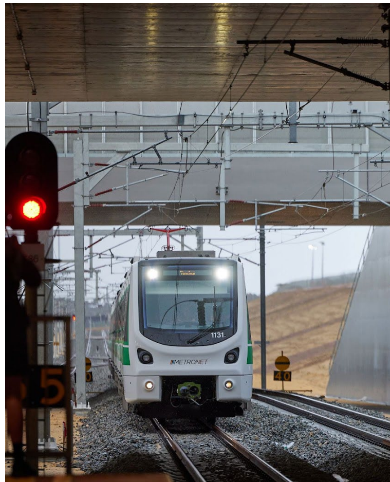
Yanchep Rail Extension — Metronet — Perth, WA, Australia.
