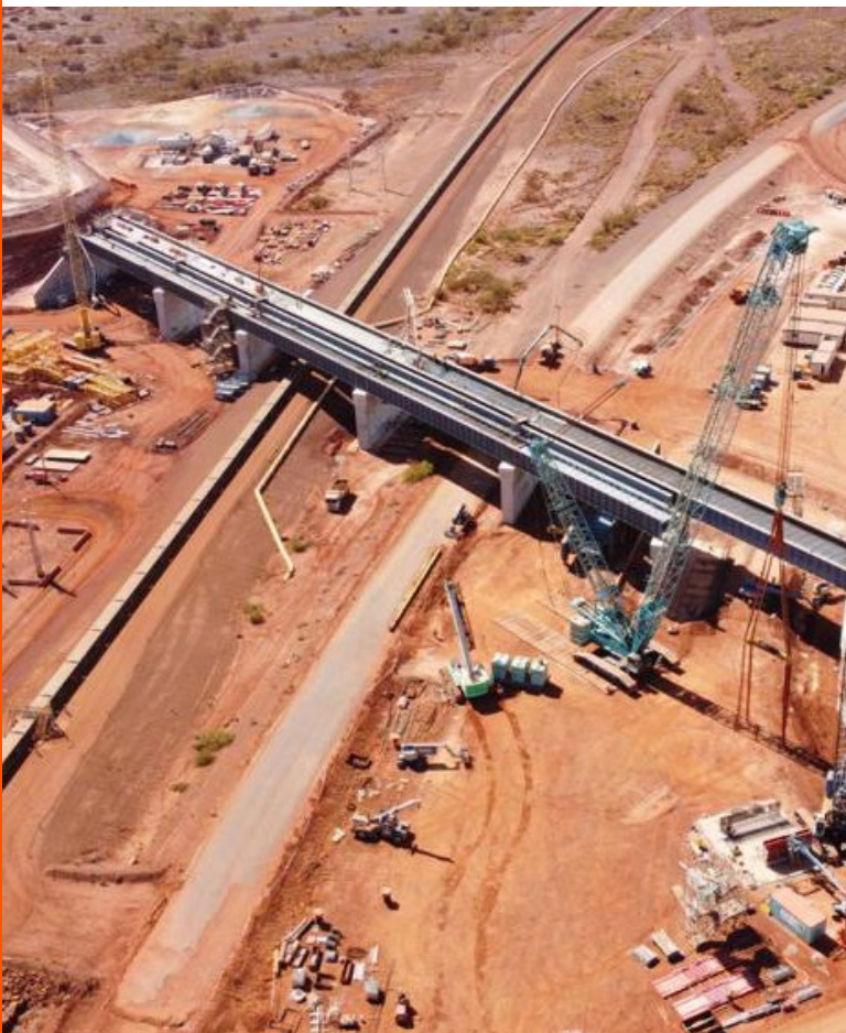
Eliwana Mine Bridges — Pilbara, WA, Australia.
