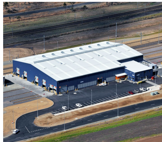
Nebo Train Maintenance Facility — Nebo, QLD, Australia.
