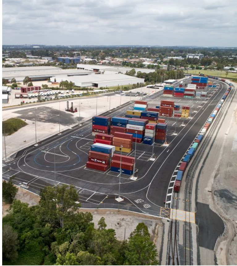
St Marys Intermodal Facility — Sydney, NSW, Australia.
