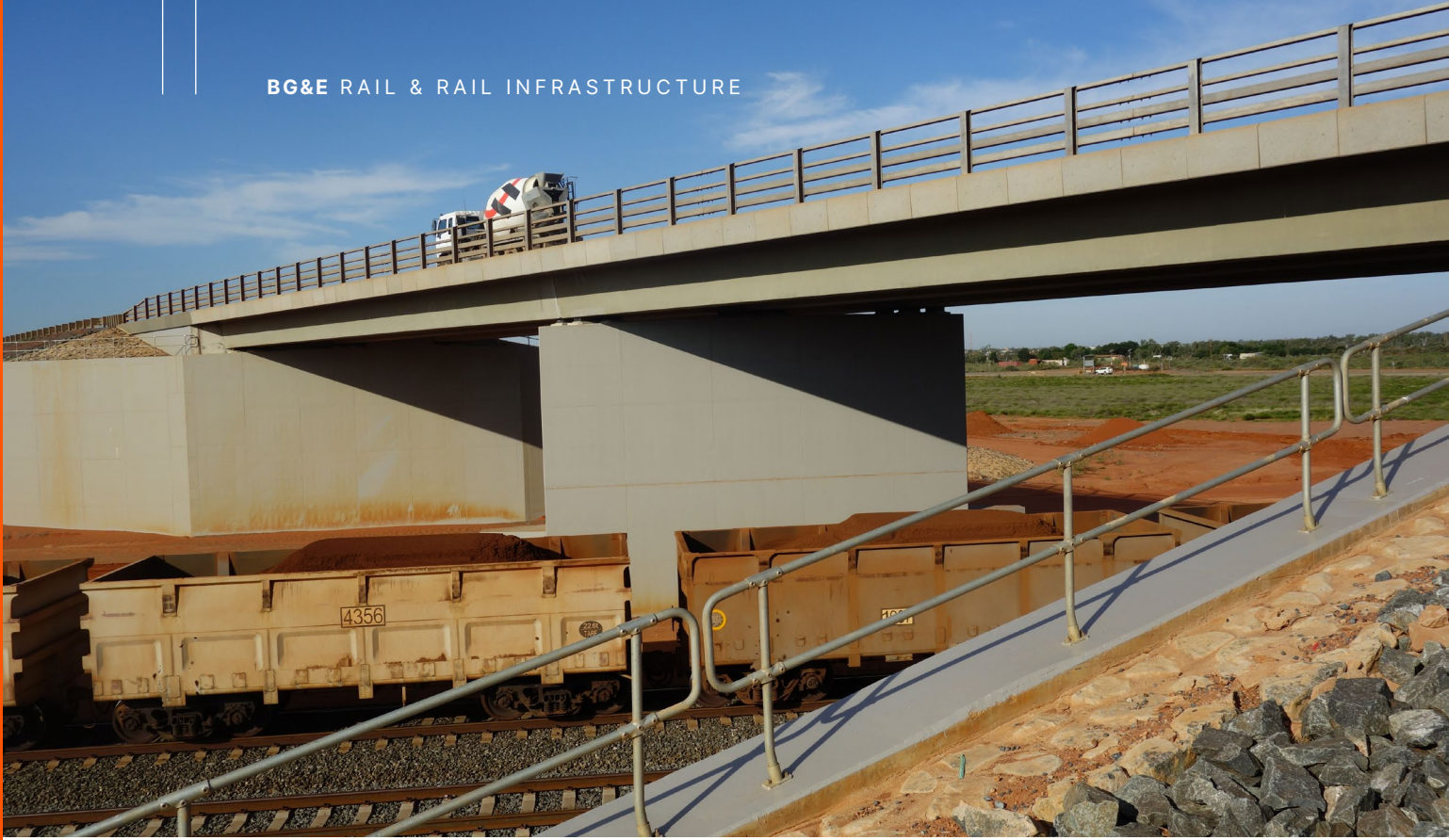
Great Northern Highway Fortescue Metals Group Solomon Road Over Rail Bridge — Pilbara Region, WA, Australia.
