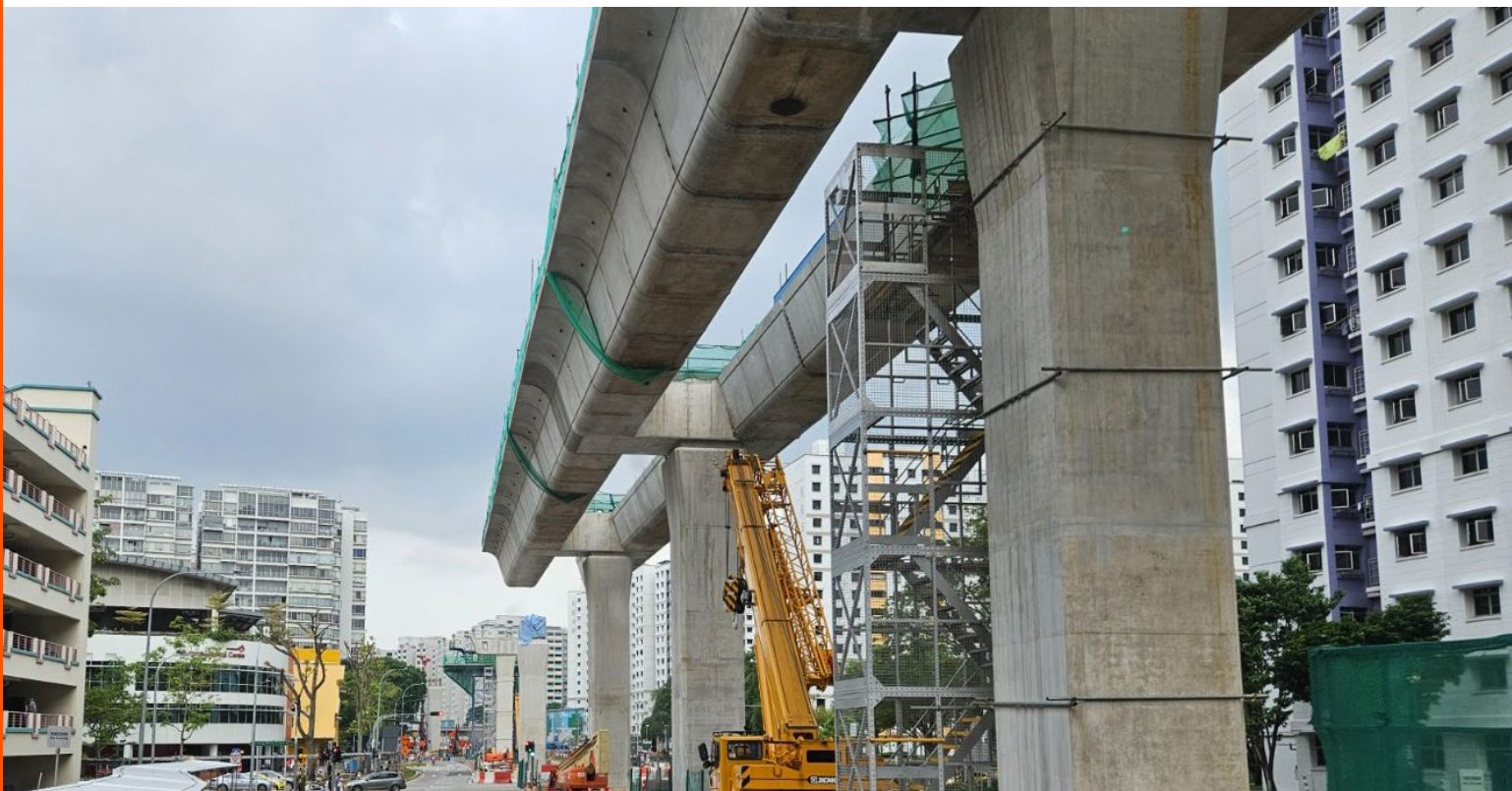
JRL 105 & 106 Rail Viaduct — Singapore, South East Asia.
