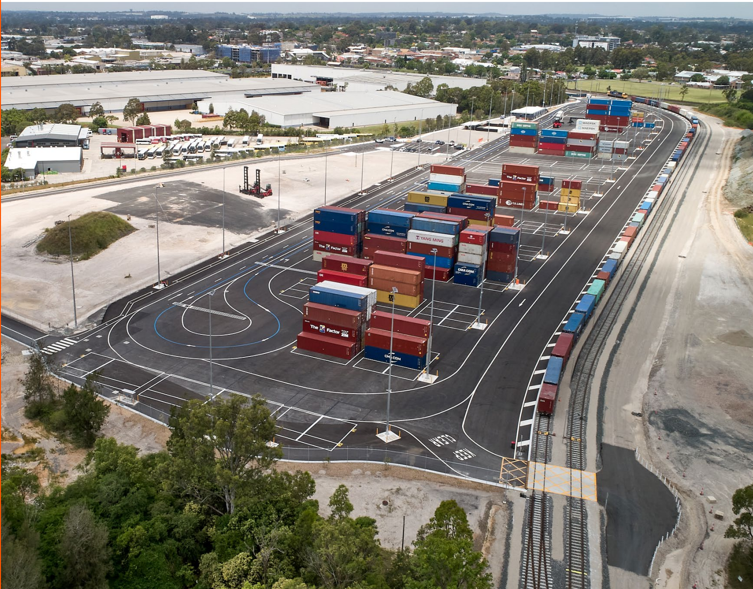
St Mary's Freight Hub — Sydney, NSW, Australia.
