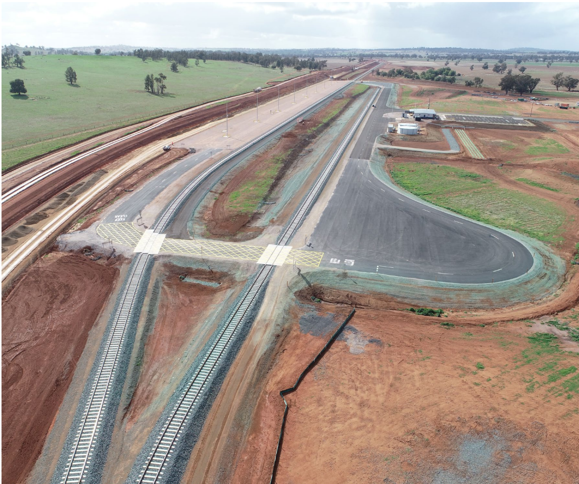
Parkes National Logistics Hub — Parkes, NSW, Australia.
