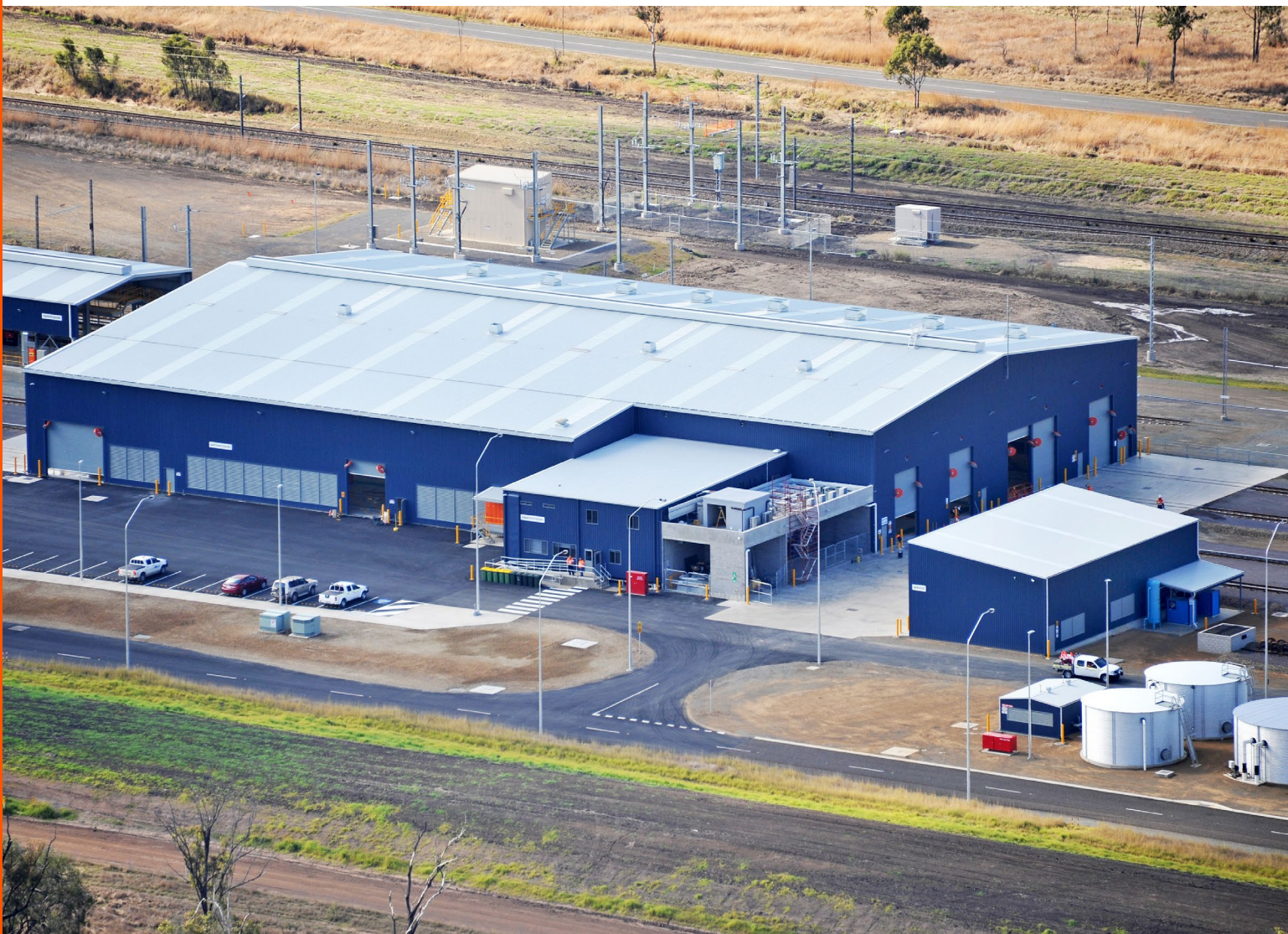
Nebo Train Maintenance Facility — Brisbane, QLD, Australia.
