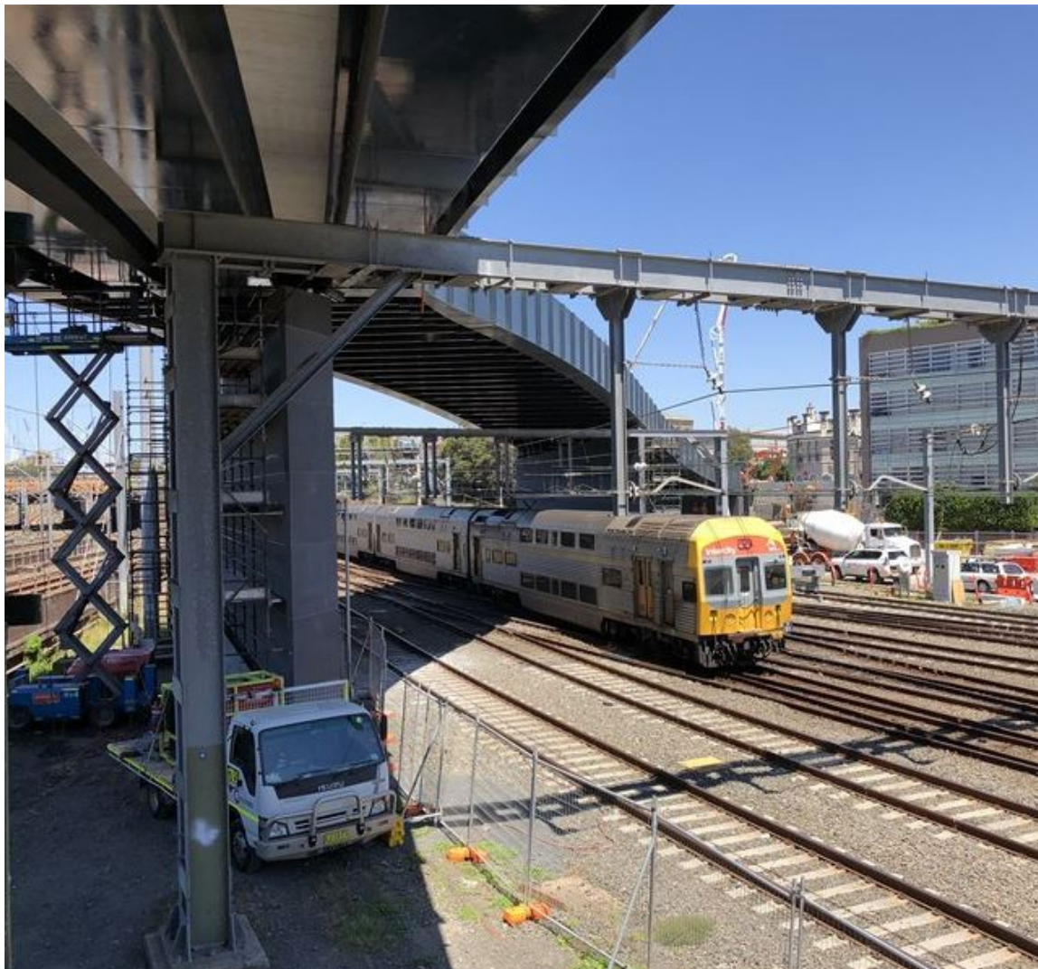
Sydney Yard Access Rail Bridge — Sydney, NSW, Australia.
