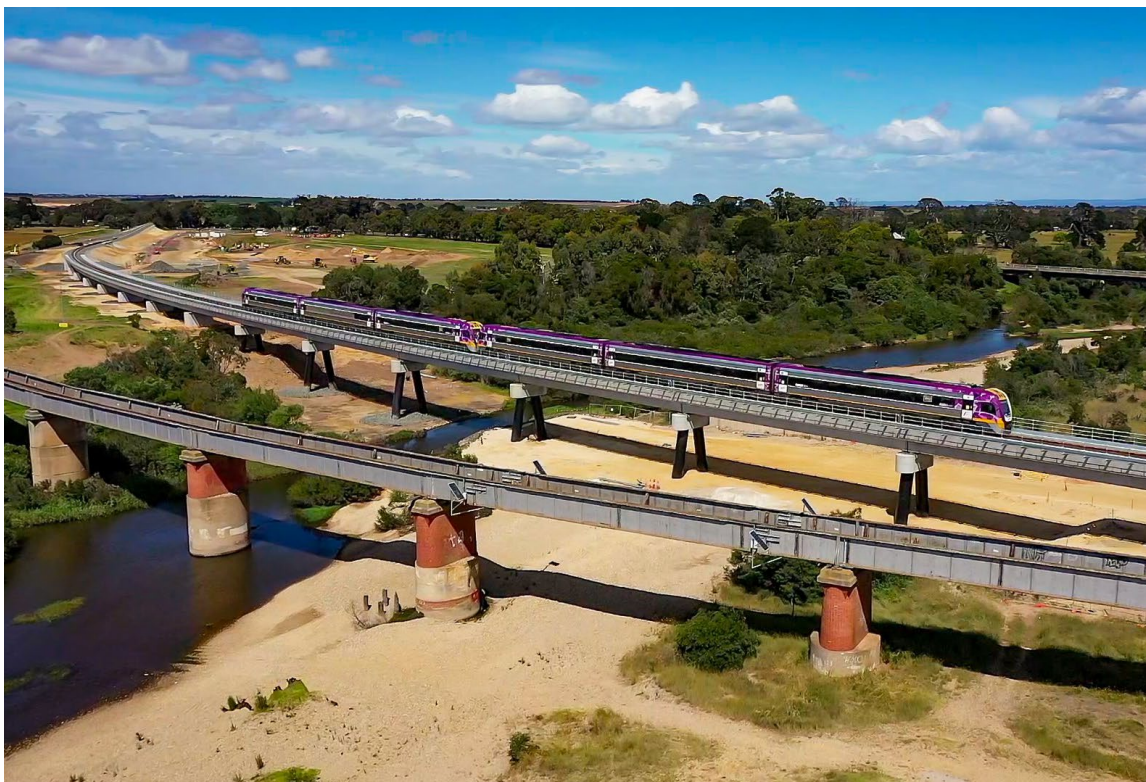
Avon River Bridge — Stratford, VIC, Australia.
