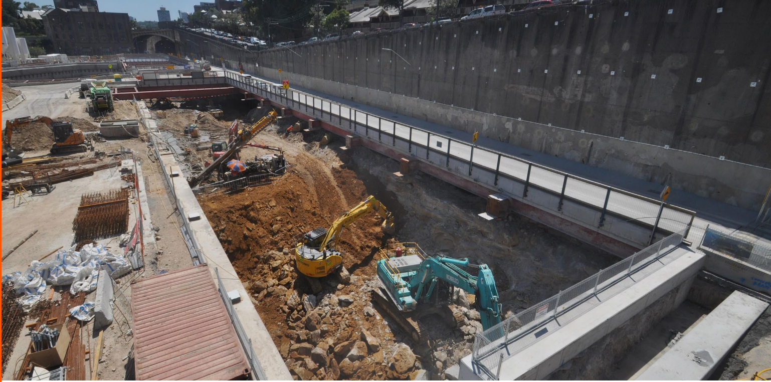
Sydney Metro — City & Southwest: Tunnel Station Excavations (TSE) — Sydney, NSW, Australia.
