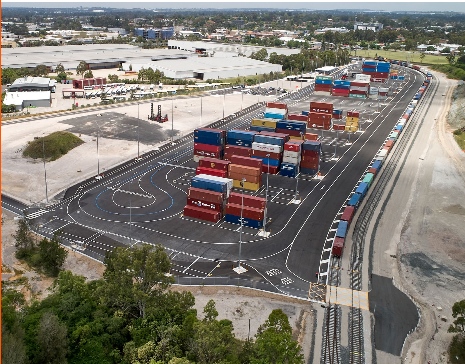
St Mary's Freight Hub — Sydney, NSW, Australia.
