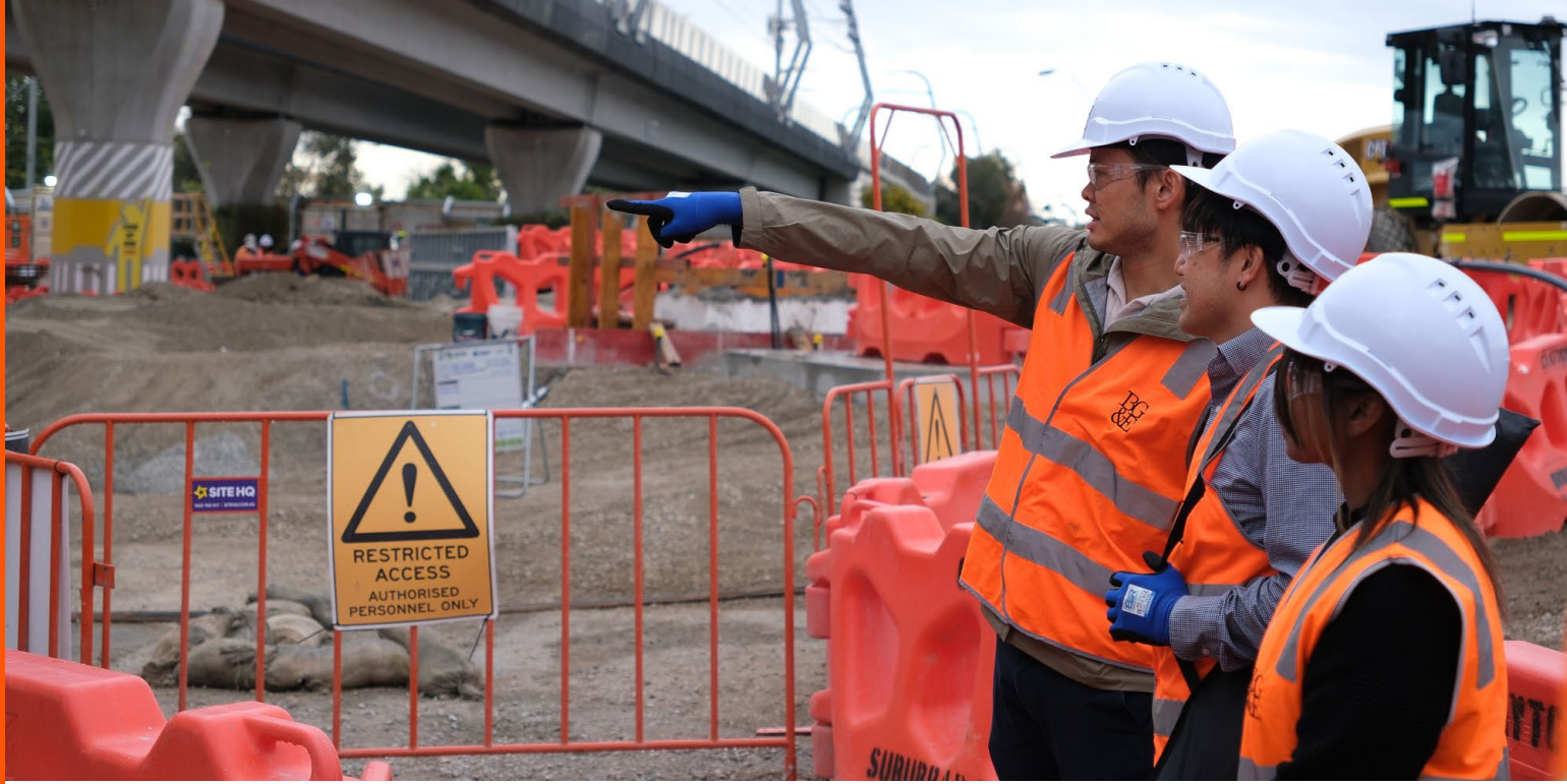
SRL East — Tunnels South (Work Package C) — Melbourne, VIC, Australia.
