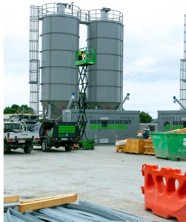
SRL East — Tunnels South (Work Package C) — Melbourne, VIC, Australia.
